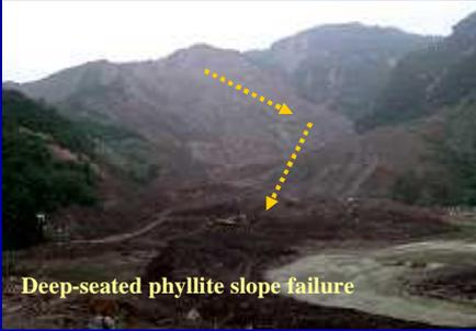
Deep-seated phyllite slope failure
