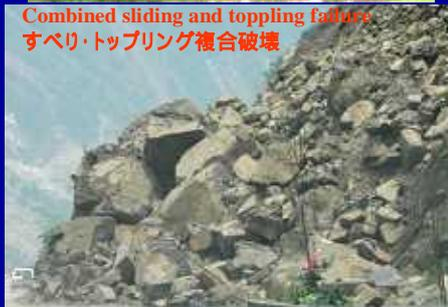
Combined sliding and toppling failure
