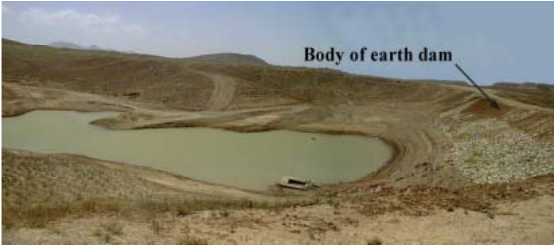
Figure 5. 8 General view of the small earth dam located northwest of Abdarreah village
