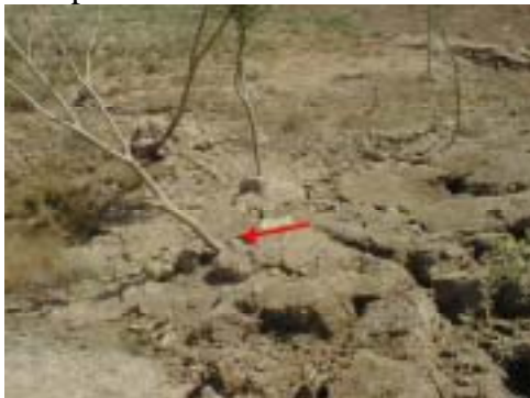
Figure 5.16. The movement of trees indicating lateral displacement of ground
