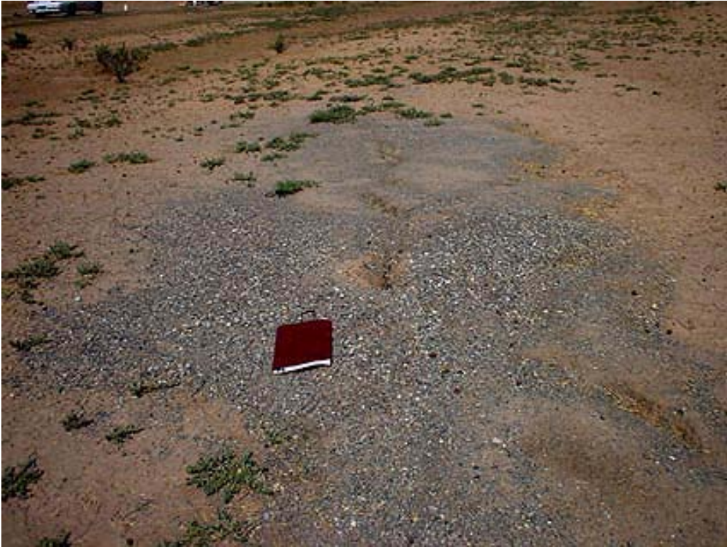
(a) Liquefied gravels
