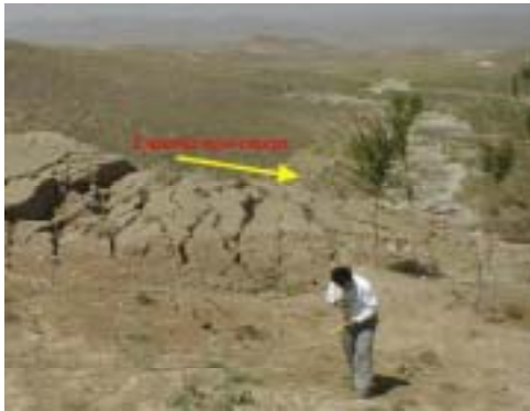
Figure 5.15. Slumping of the left bank of river at upstream side
