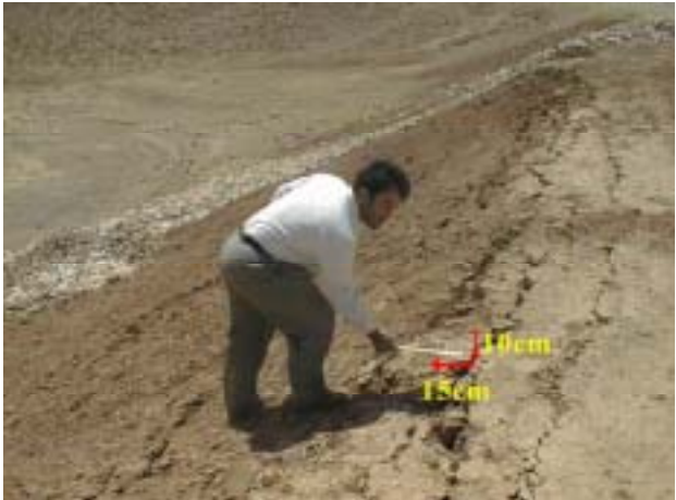
Figure 5.11. Instabilities at down stream slope
