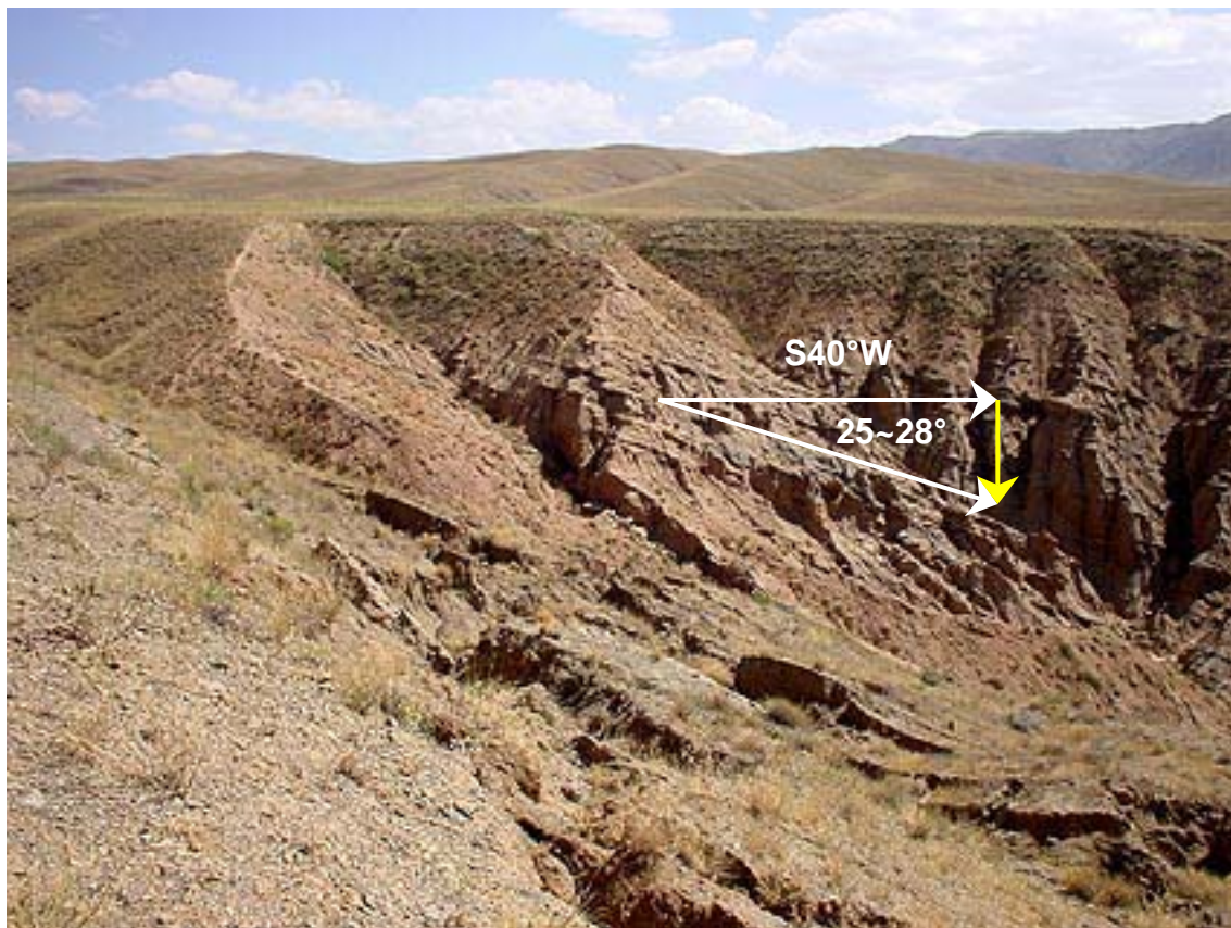
Figure 5.1 Rockslide in the foreground and Stratified structure of the rock
