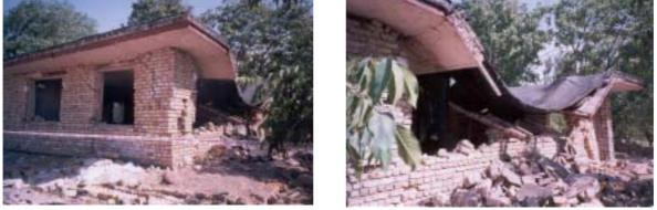
Figure 4.2 Collapse of a URM structure (Abiz)
