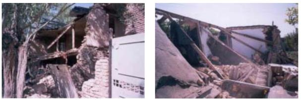
Figure 4.3 Newly constructed URM structure (Esfad)
