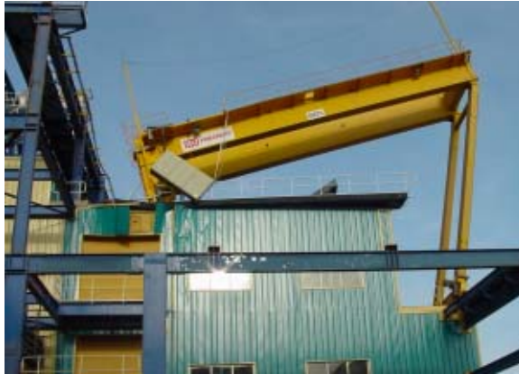
Photo 5.2.8 Gantry crane fell down
