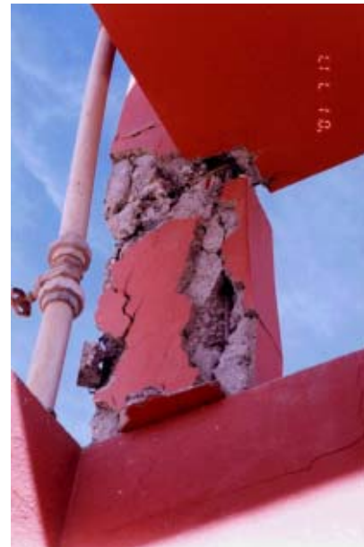
Photo 5.6 Elevated water tank at a residential building, Tacna.
