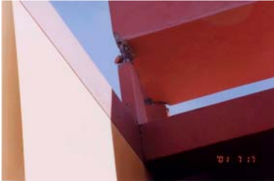
Photo 5.5 Elevated water tank at a residential building, Tacna
