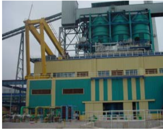
Photo 5.2.9 Crane were used for maintenance of turbine room
