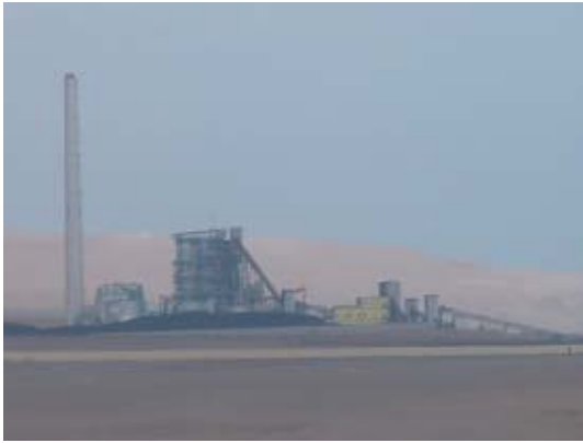
Photo 5.2.1 View of the power plant
