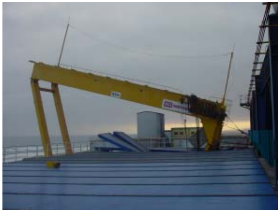
Photo 5.2.10 Crane kicked down the removable roof panels
