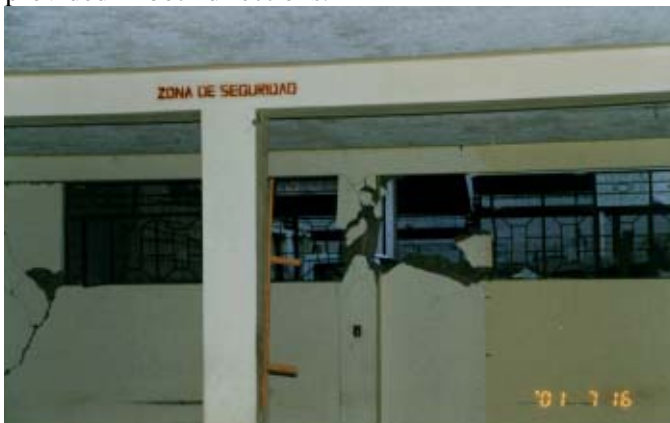
Photo 5.8. Detail of the first floor of building in Photo 5.7 .
