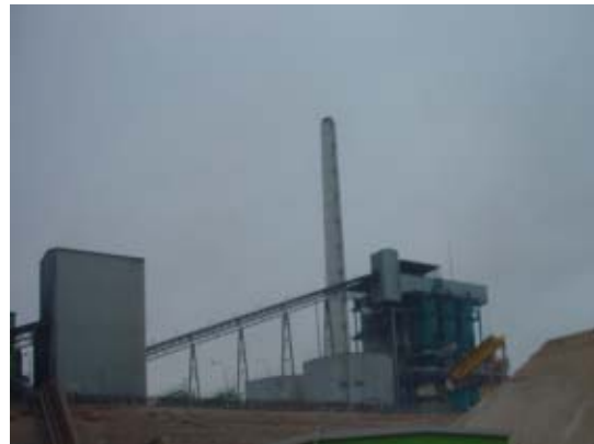
Photo 5.2.2 View of the power plant
