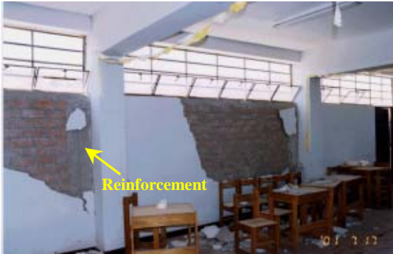
Photo 5.13. Masonry infill parapet at San Antonio School, Moquegua.
