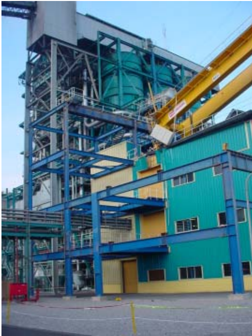
Photo 5.2.3 A view of boiler plant
