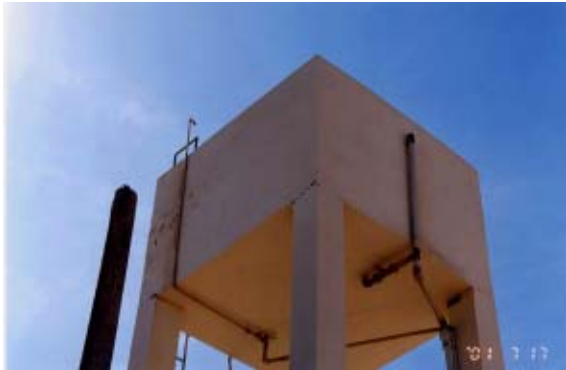
Photo 5.4 Elevated water tank, San Antonio School, Tacna
