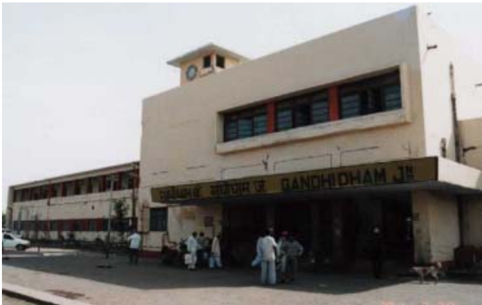
Figure 5.4 Damaged Gandhidham railway station
