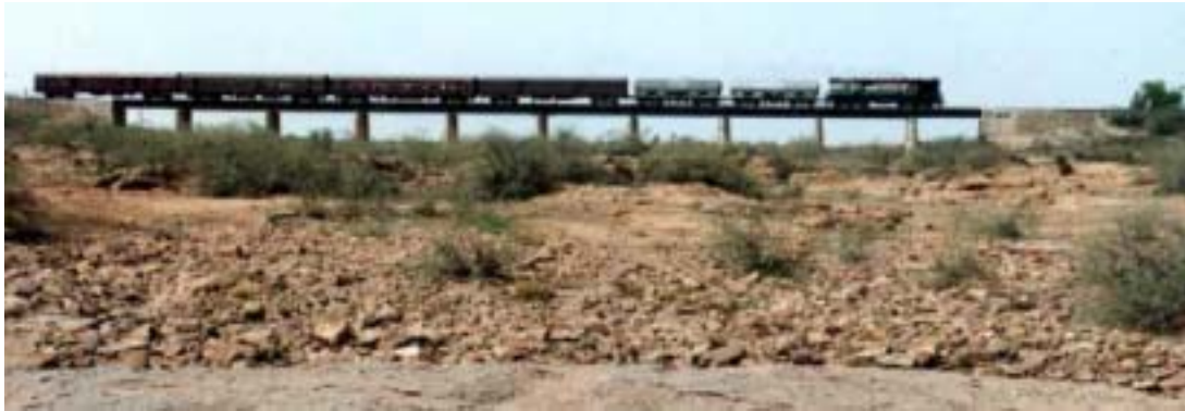
Figure 5.9 Non-damaged railway bridge on Kankawati River (7km from Halvad)
