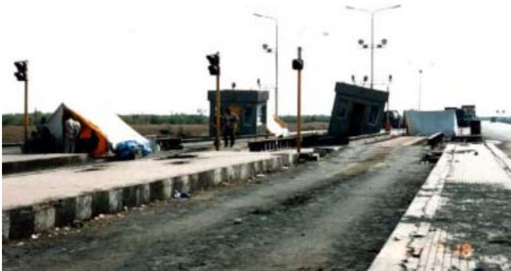
Figure 5.8 Collapsed toll gate of Highway 5A nearby Bachau
