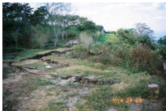
Figure 2.58. Crack at Site VI
