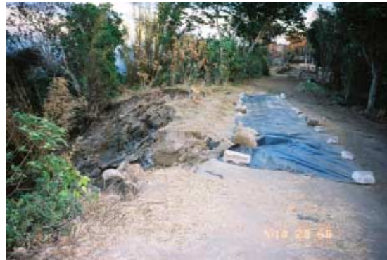
Figure 2.55. Longitudinal crack at Site III
