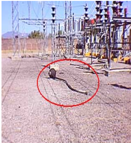
Figure 4.6. Broken insulator
