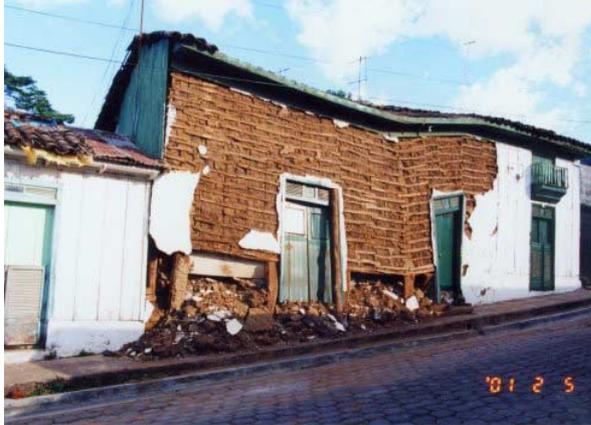
**Figure 3.28.** Damaged bahareque house with very poor foundation.
