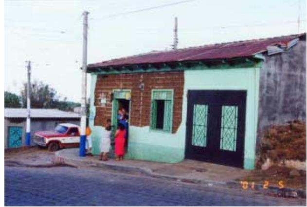
**Figure 3.29.** Bahareque house that suffered mud cover spalling.
