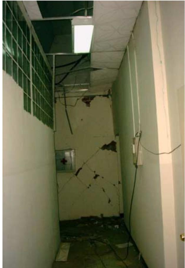
**Figure 3.36.** Typical damage in the TELECOM building (Courtesy Mr. LaFolie).
