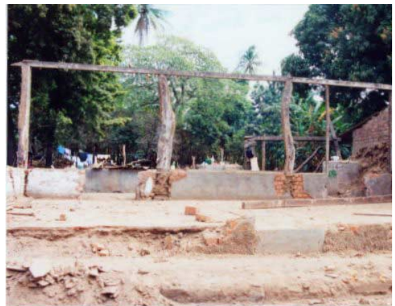
Figure 3.18. Detail of the adobe house in Figure 3.17 . Just the confining wood of one wall remained.
