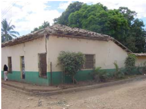
Figure 3.21. Unreinforced masonry structure. A vertical crack is observed at the connection between walls.
