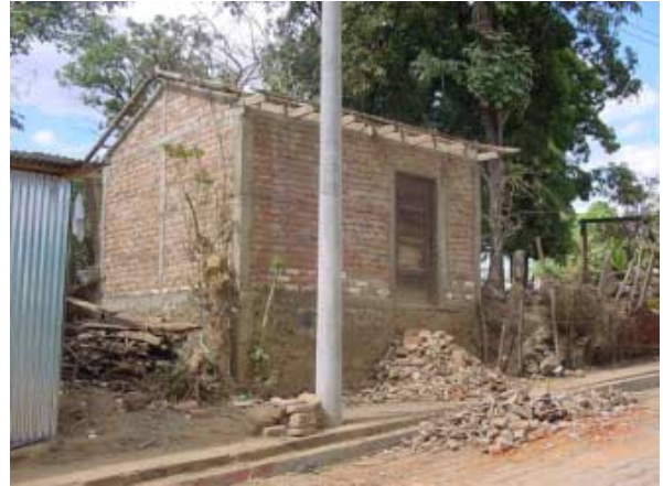
Figure 3.24. Reinforced masonry structure that did not suffer damage. However, the roof tiles felt down.
