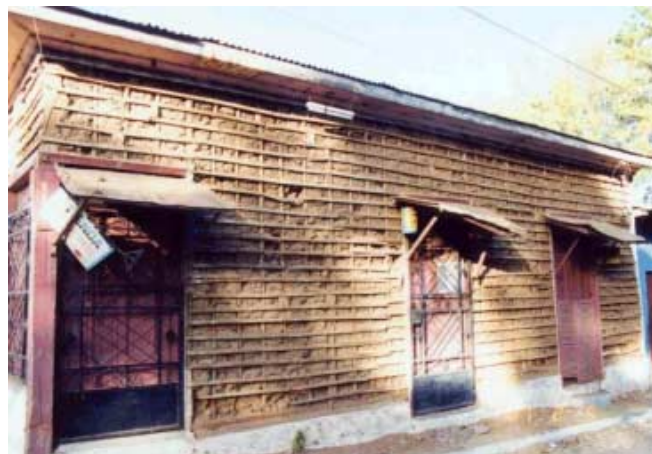
Figure 3.3. Bahareque structure which suffered mud cover spalling.
