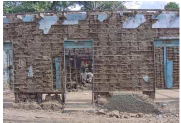
Figure 3.27. Details of the walls of the house in Figure 3.26 . Notice the poor foundation detail.
