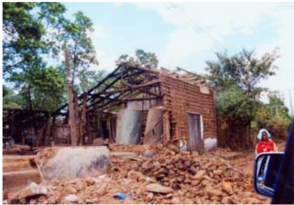
Figure 3.19. Collapsed bahareque house.
