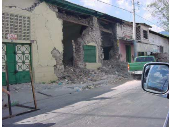
Figure 3.2. Typical adobe house that was damaged by the earthquake
