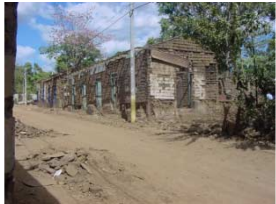
Figure 3.26. Bahareque structure damaged by the earthquake.
