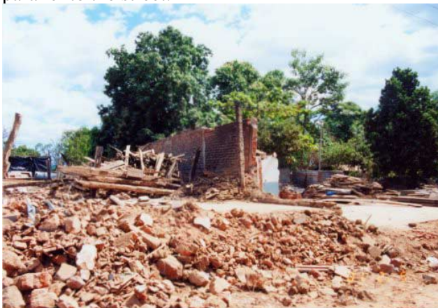
Figure 3.15. Completely collapsed adobe house.
