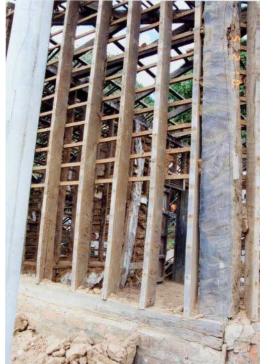
Figure 3.12. Bahareque structure that suffer mud spalling.
