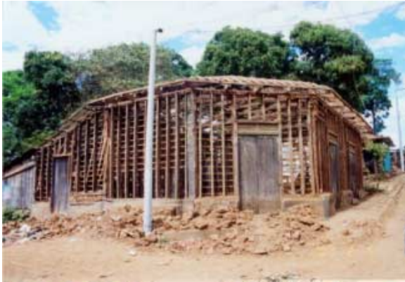
Figure 3.12. Bahareque structure that suffer mud spalling.
