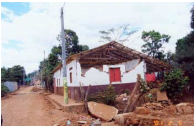
Figure 3.14. Unreinforced masonry house partially collapsed. The walls perpendicular to the street (~NE-SW direction) failed out-of-plane. The roof restrained the displacements of the top of the wall parallel to the street.
