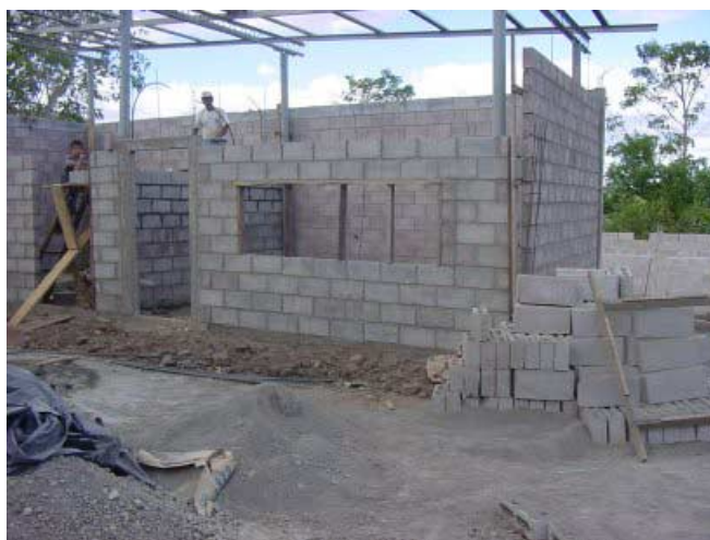
Figure 3.1. Reinforced masonry house with concrete blocks
