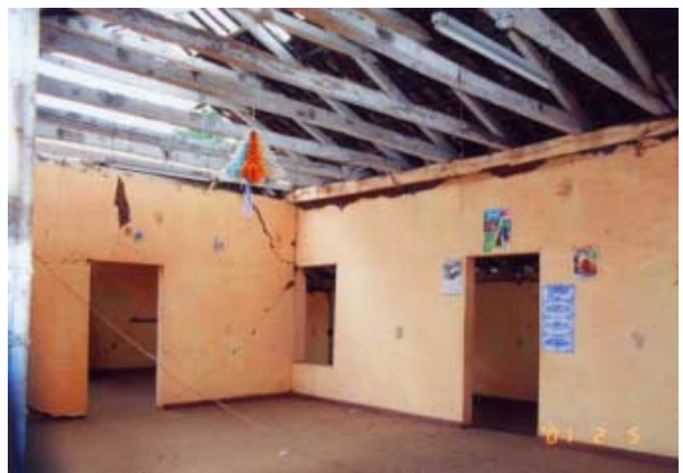
Figure 3.22. Interior of the building shown in Figure 3.21 . The wall exhibits diagonal cracking.
