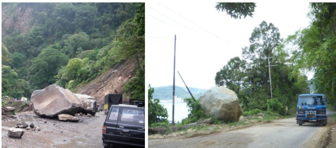
Figure 6.2: Roadway damage due to rock falls
