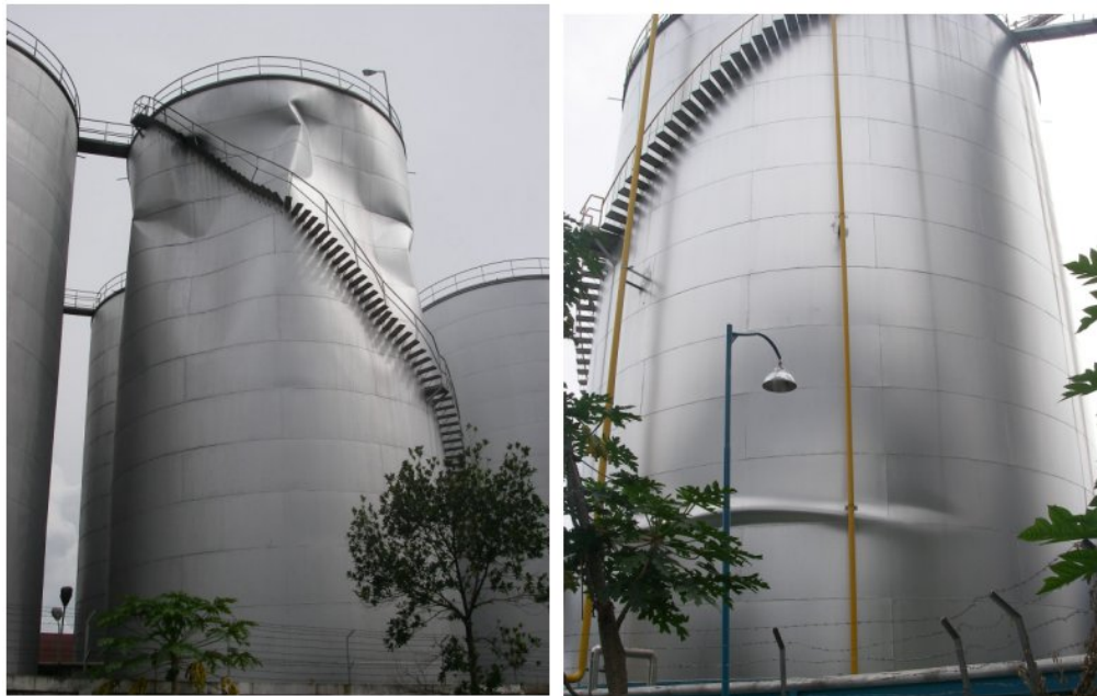
Figure 5.15: Views of buckled tanks at Teluk Bayur port
