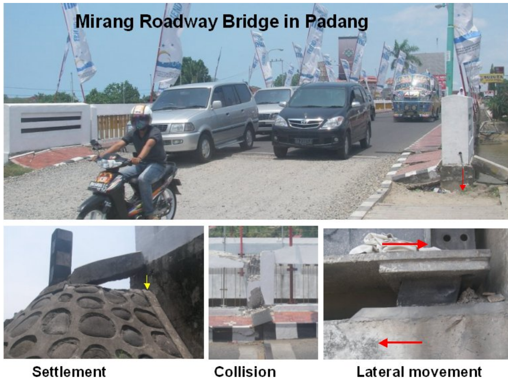
Figure 5.7: Damage to Mirang roadway bridge in Padang
