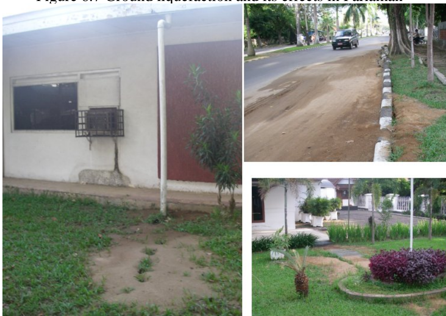
Figure 6.8 Ground liquefaction in Padang
