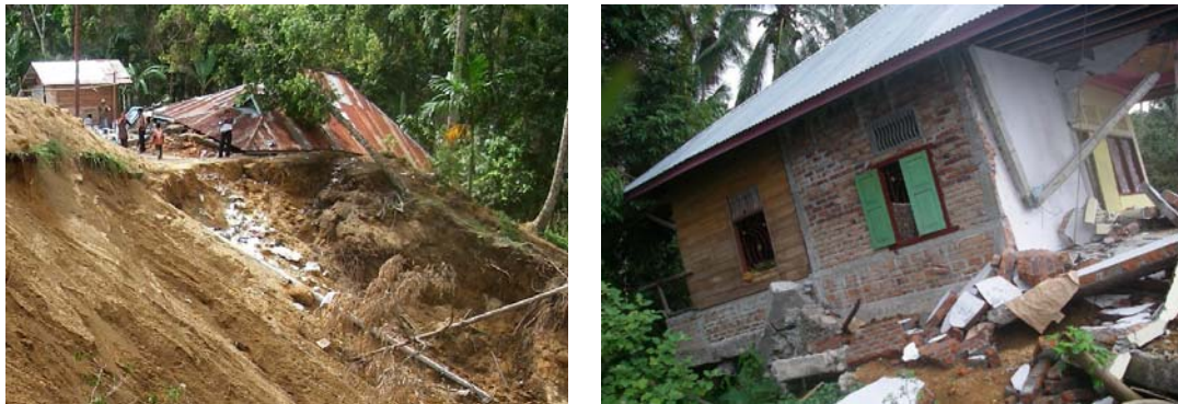
Figure 5.3: Collapsed or heavily damaged buildings due to foundation failure by landslides
