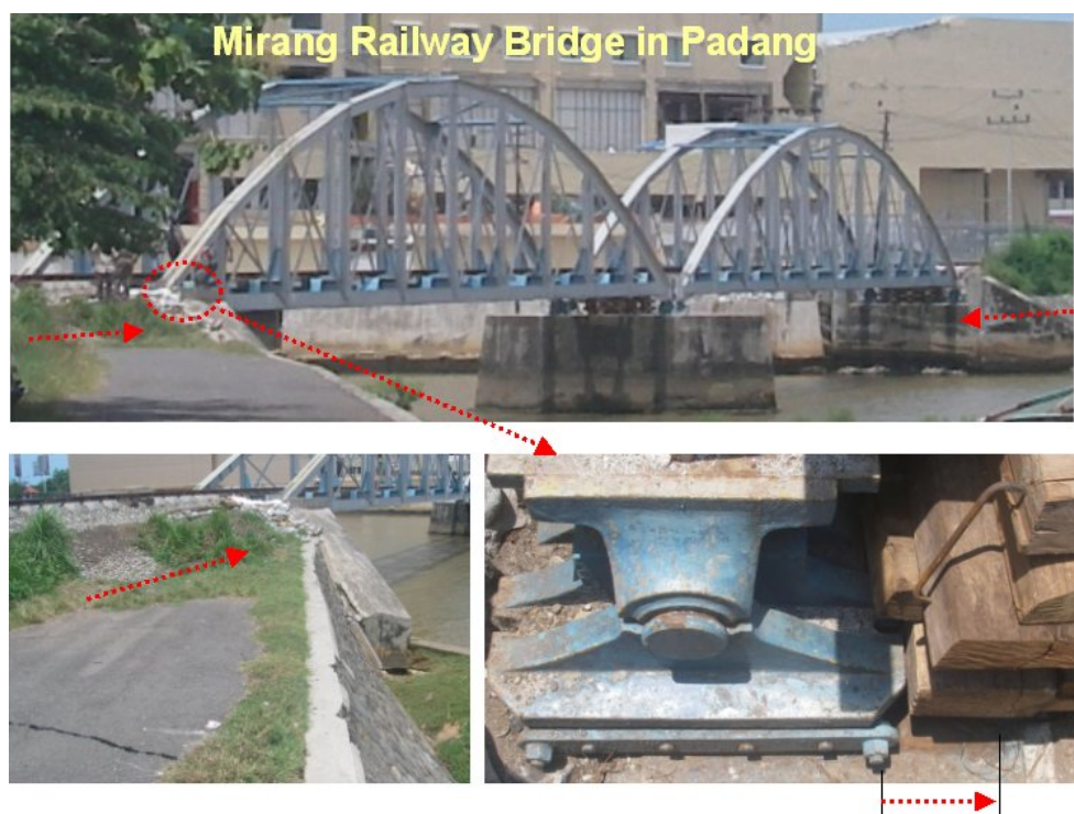
Figure 5.6: Damage to Mirang railway bridge in Padang
