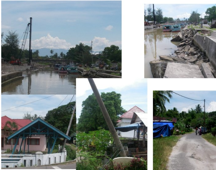
Figure 6.7 Ground liquefaction and its effects in Pariaman
