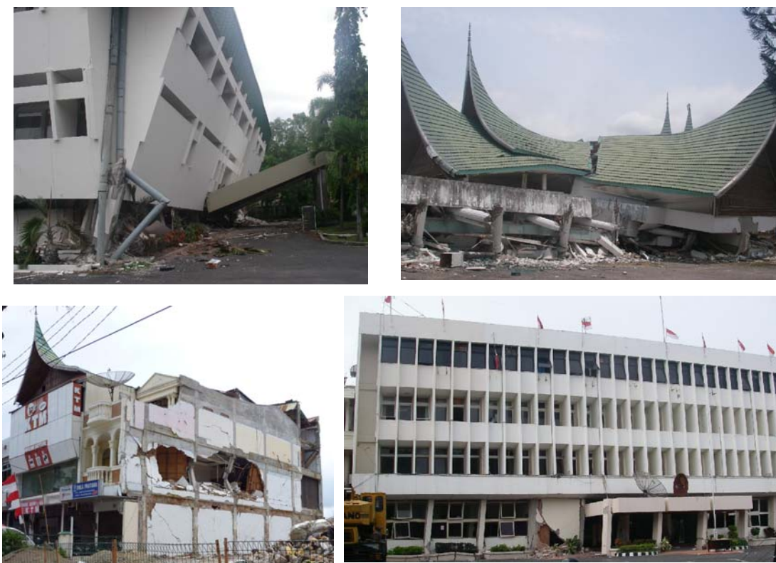
Figure 5.4: Collapsed or heavily damaged RC buildings
