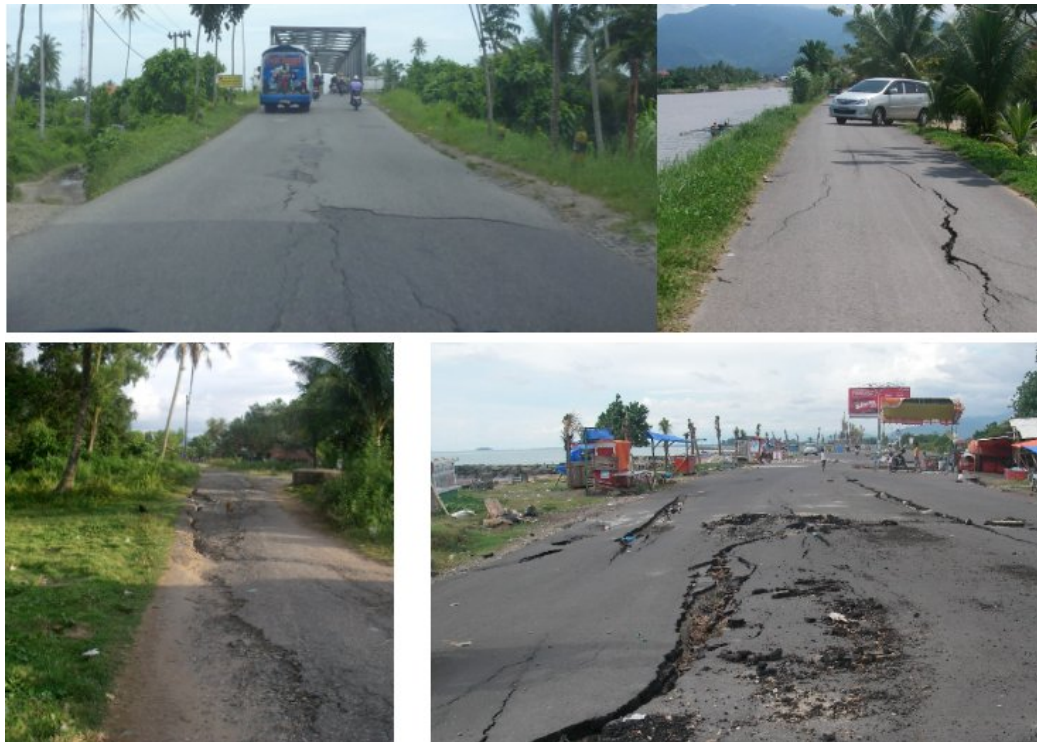
Figure 6.6: Views of some embankment failures in the epicentral area
