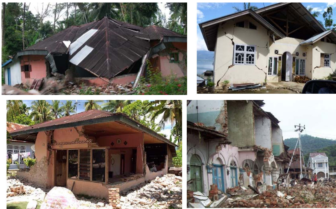
Figure 5.2: Collapsed or heavily damage masonry buildings
