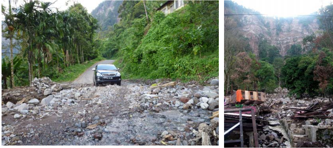
Figure 6.5: Debris flow induced damage due to the breach of landslide dams
