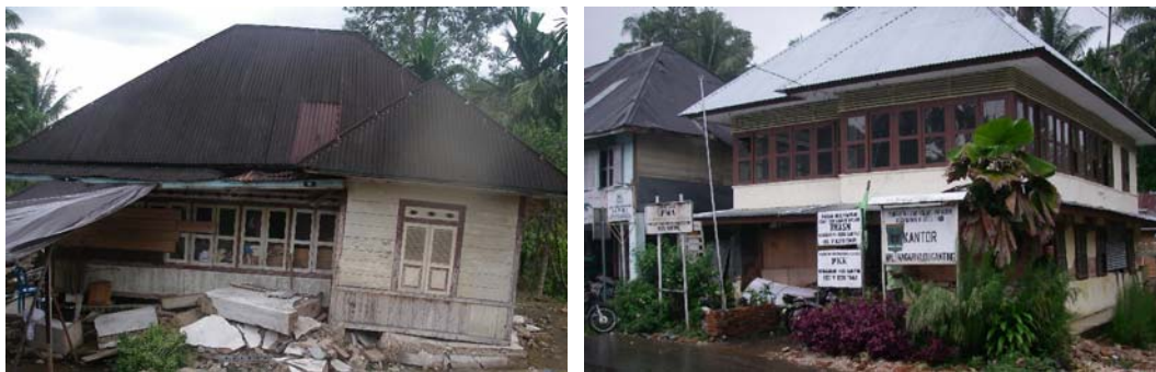
(a) Damaged due to foundation failure
