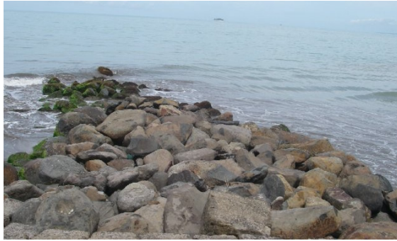
(a) Subsidence of wave break at Pariaman
