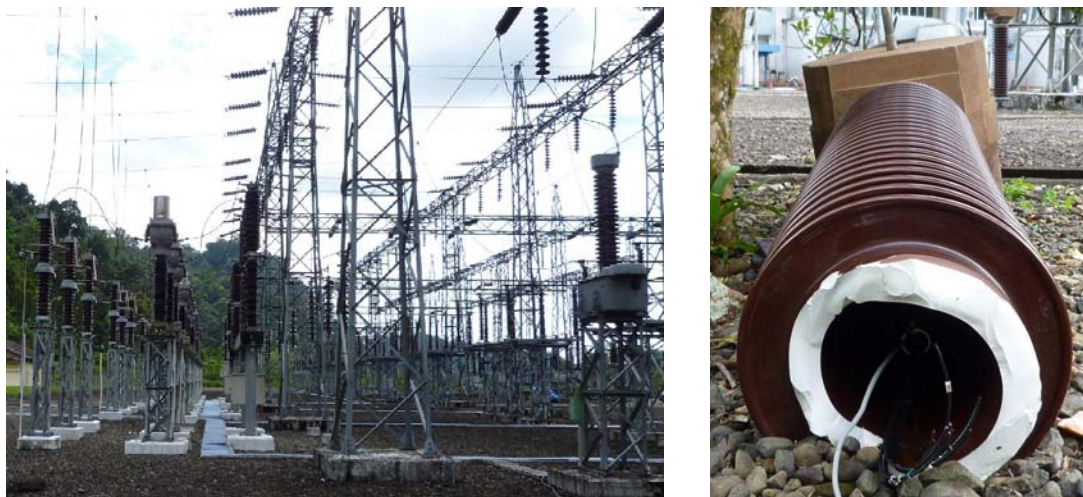
Figure 5.12: A view of Maninjau sub-station and broken ceramic isolator.
