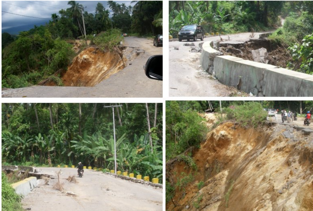
Figure 6.1: Roadway damage due to slope failures in Padang Alai
