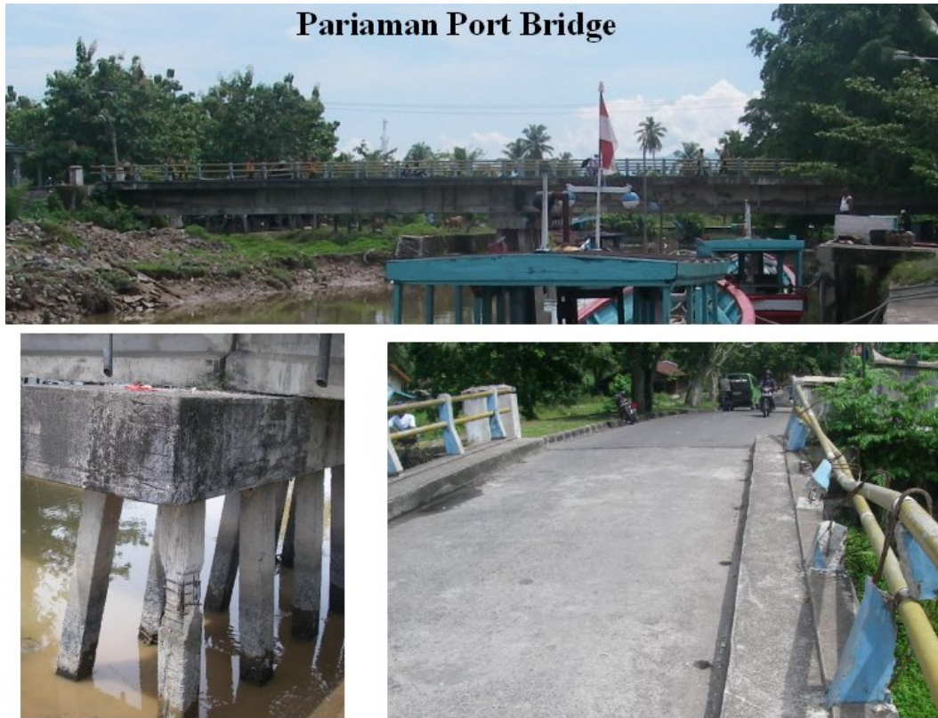
Figure 5.9: Slight damage to piers and railings
