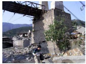
**Fig. 6**, Suspention bridge near Balakot bridge: The right tower was cut off and shifted towards downstream side.
