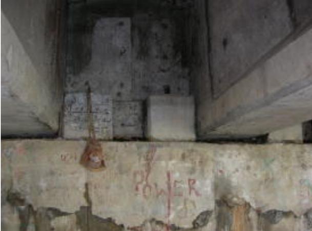
Photo 11.14 Slight Damage to Shear Keys
