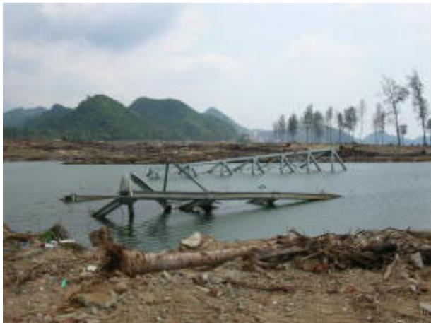
Photo 11.19 Washing out of Steel Truss
