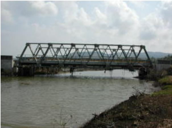
Photo 11.15 Steel Truss Bridge without Damage
