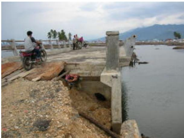
Photo 11.9 Lateral Displacement of Deck
