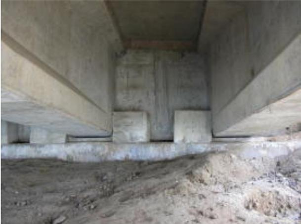
Photo 11.12 Concrete Block Shear Keys
