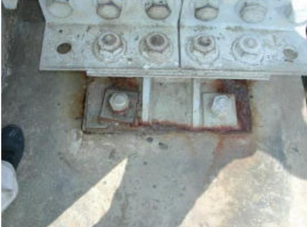
Photo 11.16 Steel Bearing Supports
