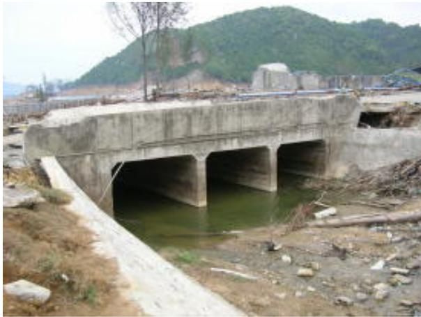
Photo 11.22 Concrete Box Culvert Bridge
