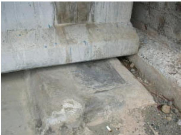
Photo 11.7 Lateral Displacement of Deck
