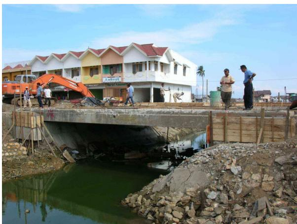
Photo 11.1 Repair of Washed-out Girder Bridge
