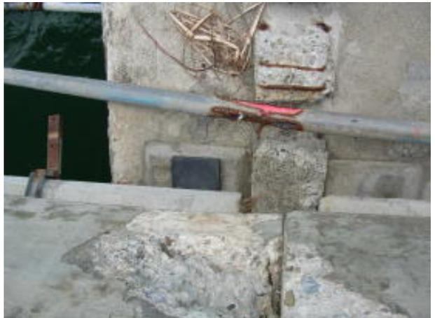
Photo 11.8 Rubber Sheet Type Bearing and Lateral Displacement at Bearing
