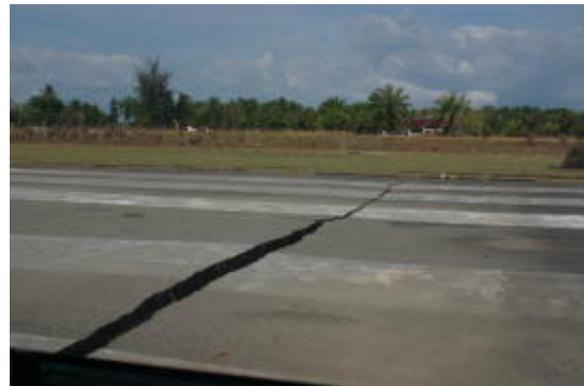
Photo 11.34 Damage of Airstrip
