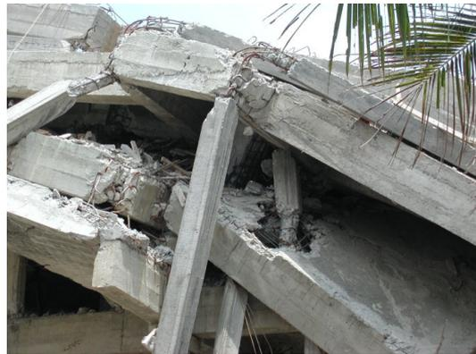
Photo 7.3(b) Collapsed or heavily damaged RC buildings
