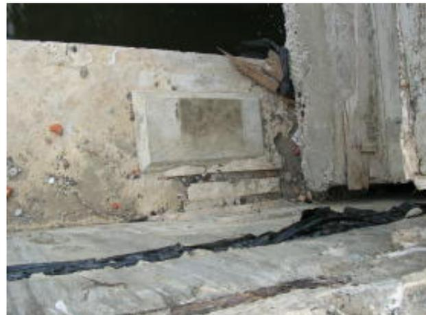
Photo 11.10 Displacement at Bearing
