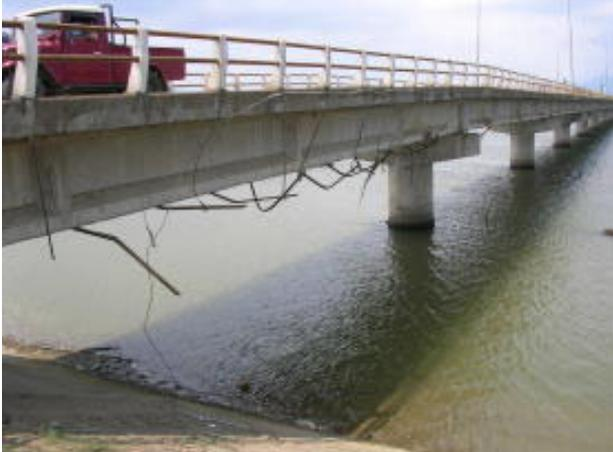
Photo 11.11 Undamaged Bridge by Tsunami
