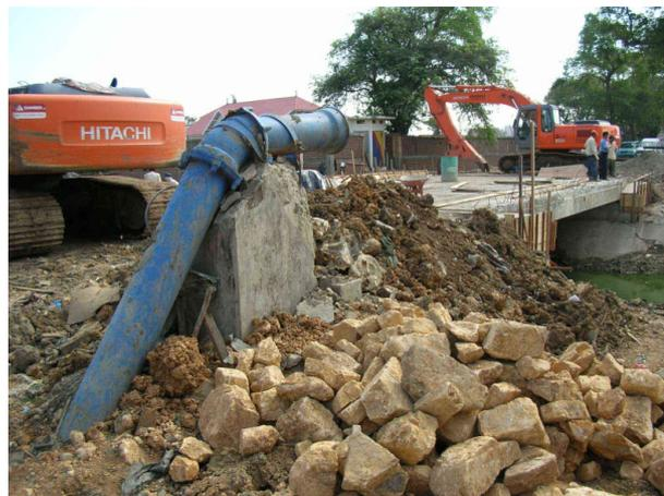
Photo 11.2 Collapse of Water Pipes
