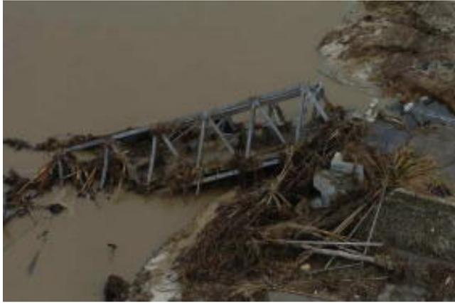
Photo 11.24 Washout of Truss Bridge (1)
