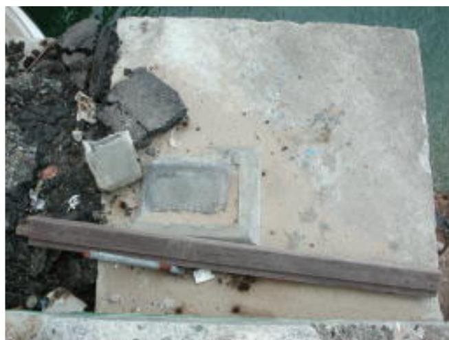
Photo 11.21 Bearing Support and Bolt to connecting Deck and Substructures
