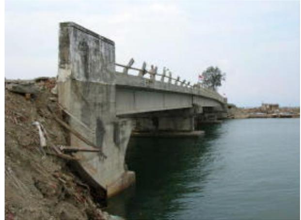
Photo 11.6 Washout Effect of Backfill Soils
