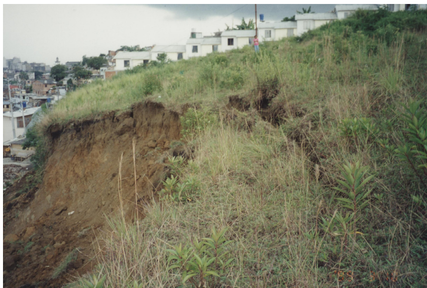
Photo 2. An example of slope failure
