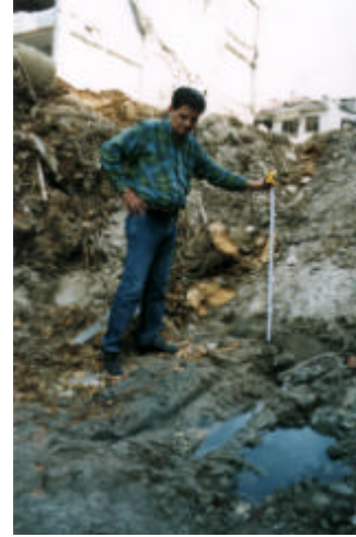
Figure 4.7 Ground conditions in the city center of Adapazar
