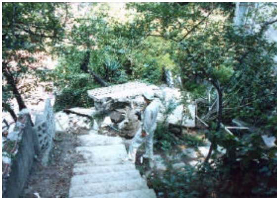
Figure 4.10 Faulting in Gölçük
