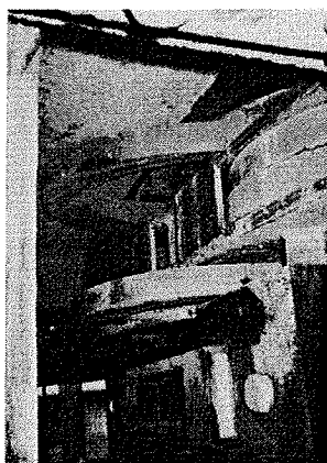
Photo 13 Energy Dissipating Elements that suffered Damage resulting from Excessive Movement of the Deck
