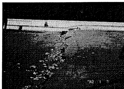
Photo 11 Shear Failure of Deck resulting from the Offset of Girder from the Pier
