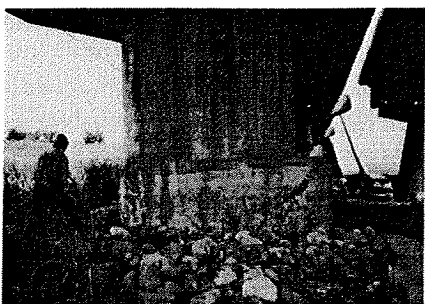
Photo 18 Shear Failure of Caisson Foundation Resulting from Fault Movement, Wu-Shi Bridge
