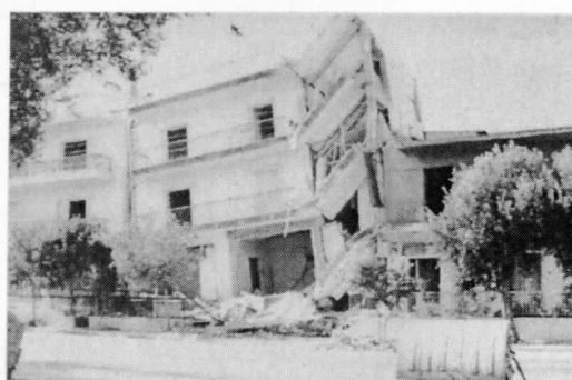
Photo 3 Damage due to pounding, Menidi.
