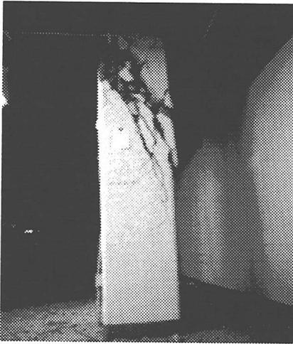
Fig.2a Collapse of a column at the upper level.
