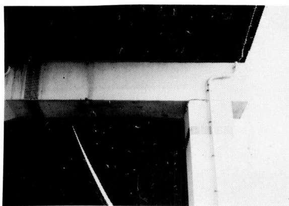
Photo 15. Crack of Beam-Column Connection (Harbor Highway)
