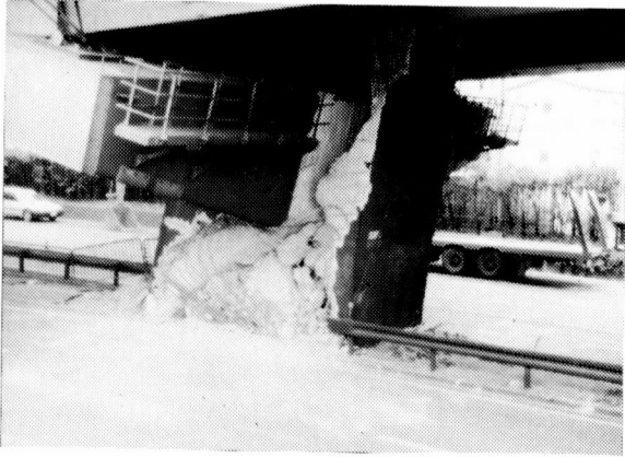
Photo 19. Shear-Failure of Concrete Pier (Hanshin Expressway, Route No.3)
