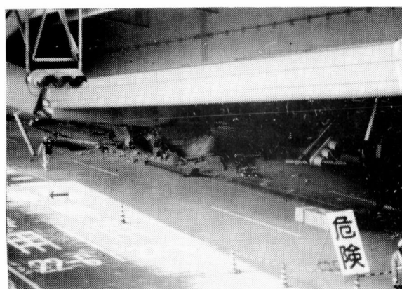
Photo 14. Collapse of Steel Pier, Tateishi Intersection (Hanshin Expressway, Route No.3)
