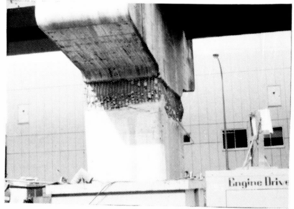
Photo 20. Damage of Concrete Pier (Harbor Highway)
