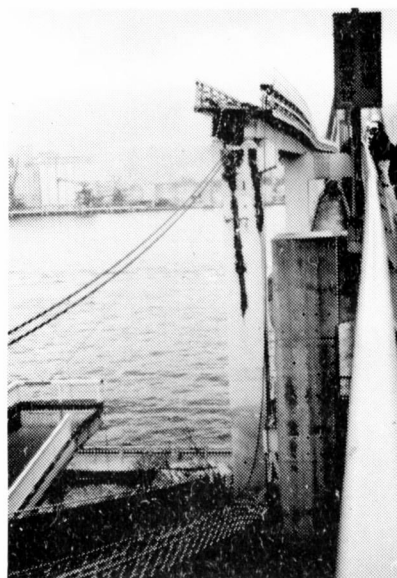
Photo 10. Fall-down of Steel Girder (Rokko Liner)
