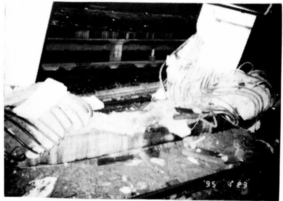
Photo 22. Failure of Center Columns (Kobe Subway)
