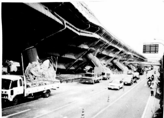
Photo 1. Roll-over of Concrete Girder Viaduct (Hanshin Expressway, Route No.3)
