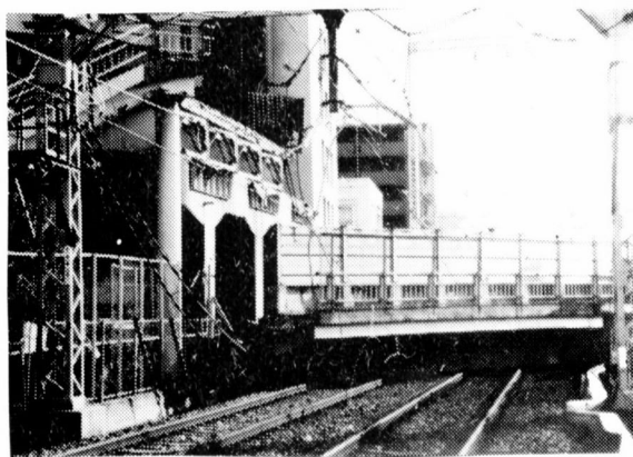
Photo 8. Fall-down of Overpass Bridge (National Road Route 171)
