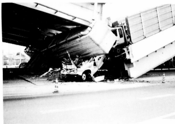
Photo 3. Collapse of Concrete Pier (Hanshin Expressway, Route No.3)
