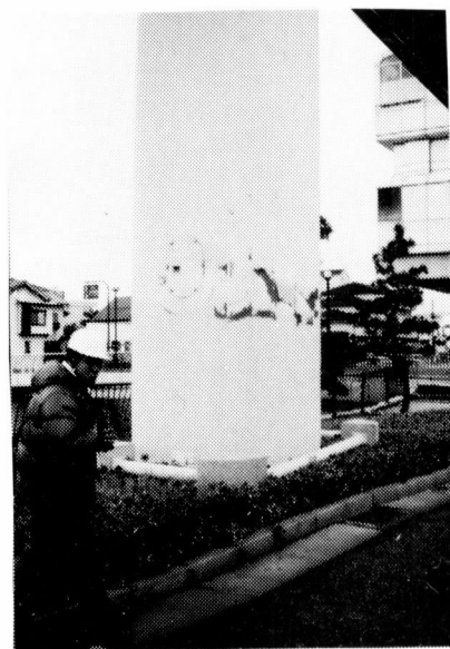
Photo 4. Buckling of Steel Pier (Rokko Liner)
