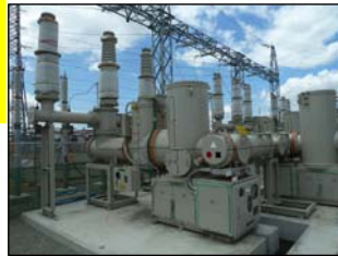
GAS INSULATED SUBSTATION
