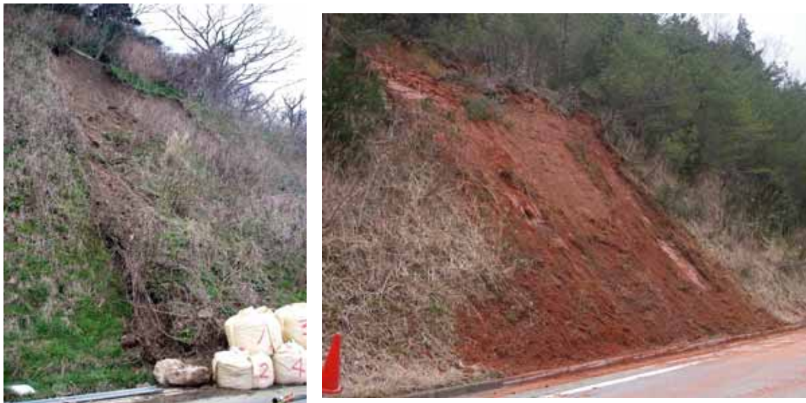
Figure 8.6: Surficial slope failures
