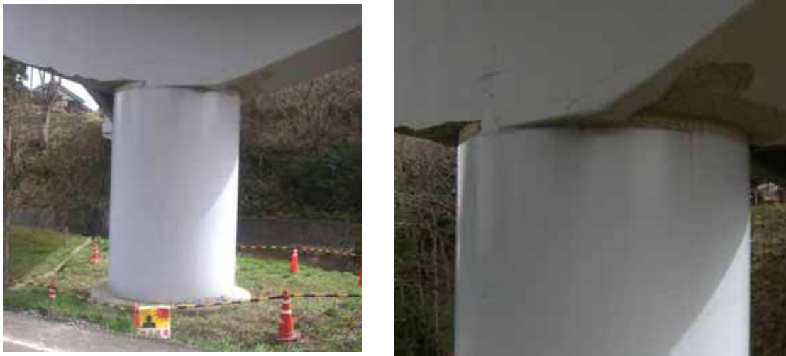
Figure 7.15: Piers with spalling
