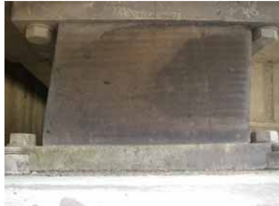
(b) strained rubber bearing (south side)
