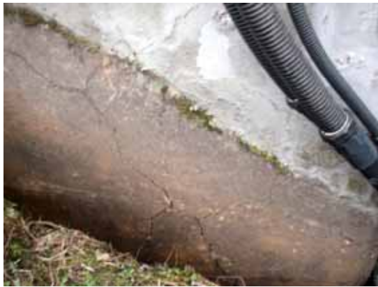
(a) Fractures and embankment separation
