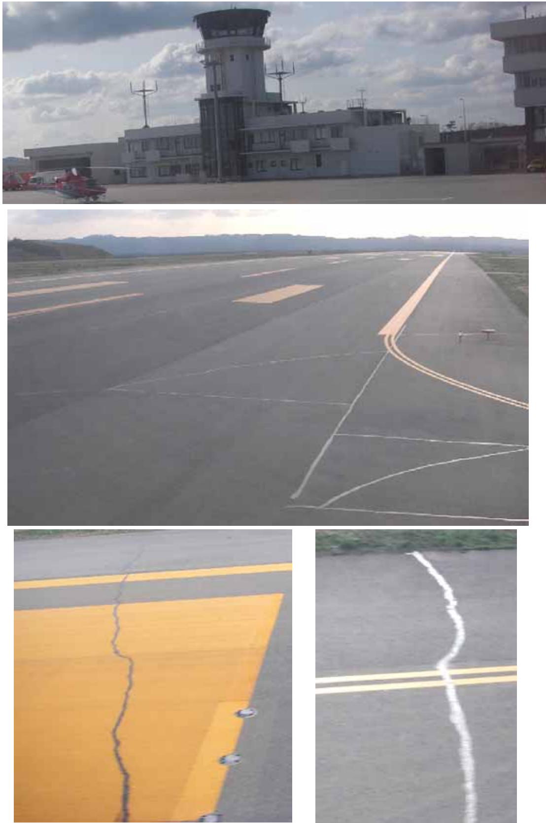
Figure 7.22: Views of non-damaged control tower and cracked runway at Noto Airport
