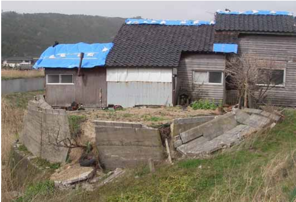
Figure 7.2: An example of damaged house built on an embankment in Monzen town
