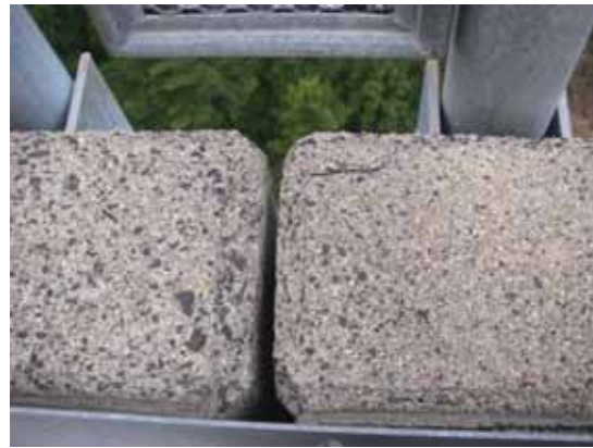
(b) fragmentation at the connection joint
