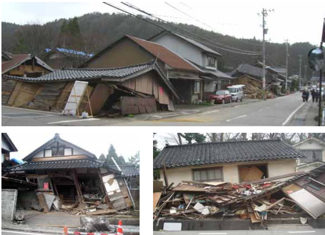
Figure 7.1: Some typical examples of collapsed or heavily damaged wooden houses
