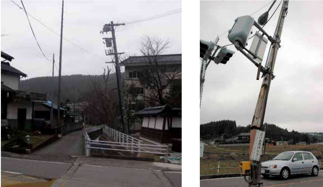
Figure 9.2: Inclined or damaged poles in Monzen town
