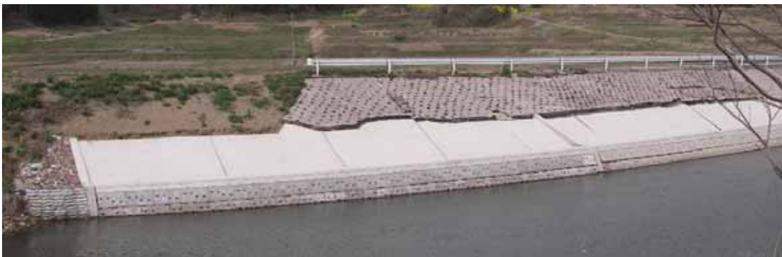
(a) Embankment failure in Toge district of Monzen town
