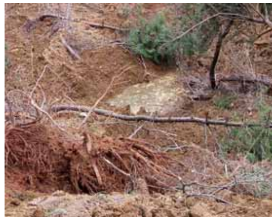
(b) waterpool at the toe of the failed embankment
