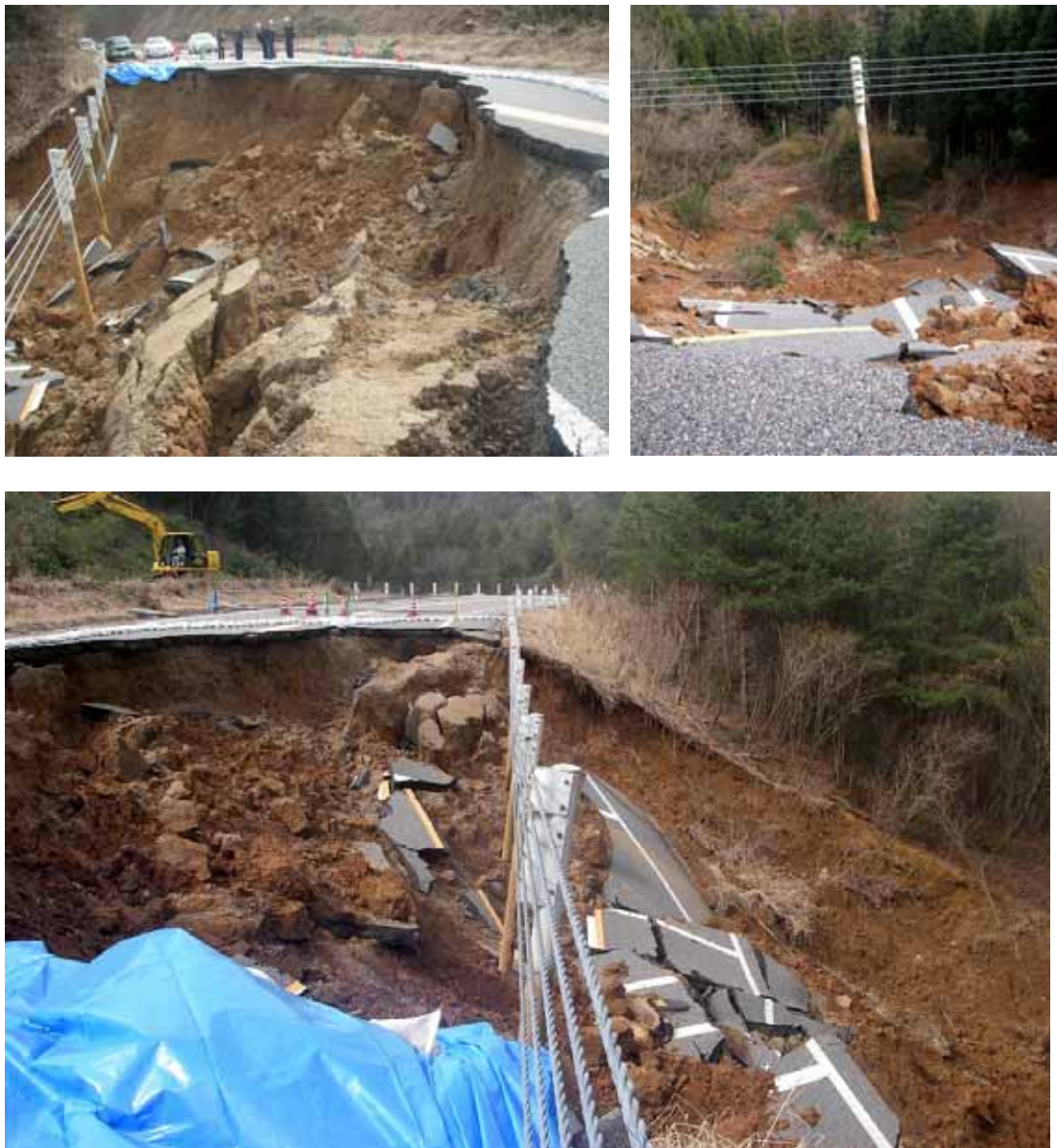
Figure 7.8: Failure of embankments of Noto Tollway
