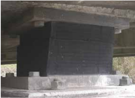
(a) Ruptured rubber bearing (north side)
