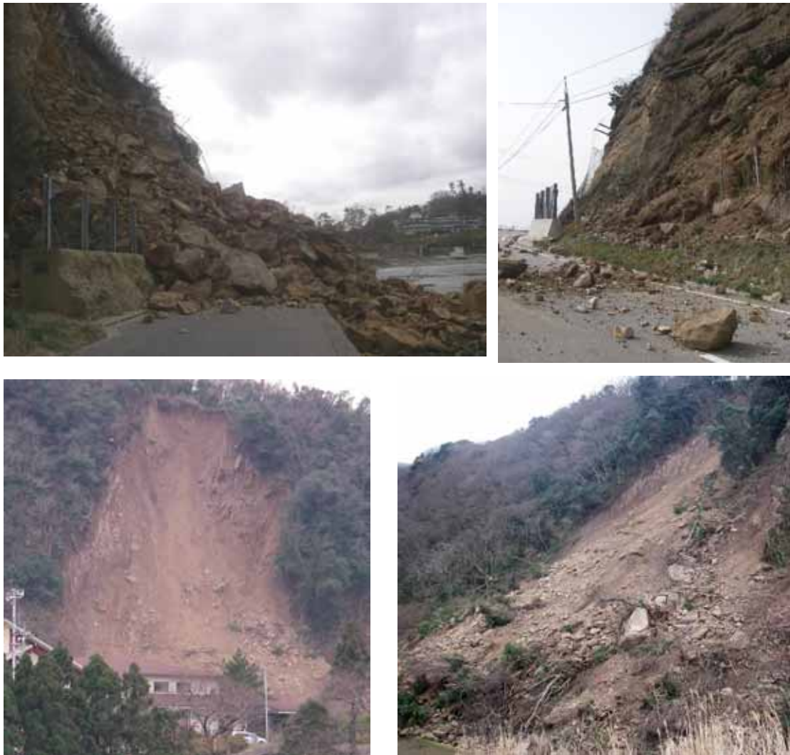
Figure 8.7: Combined sliding and toppling failure of rock slopes
