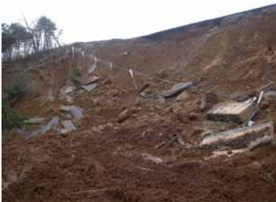
(a) Failed embankment of Noto Tollway
