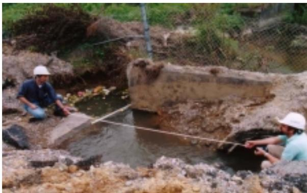
Figure 8.4 Breakage of sewage pipe crossing a main fault
