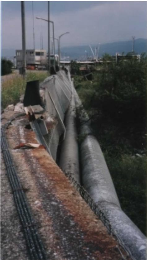
Figure 7.10 The fallen pipes from embankment wall
