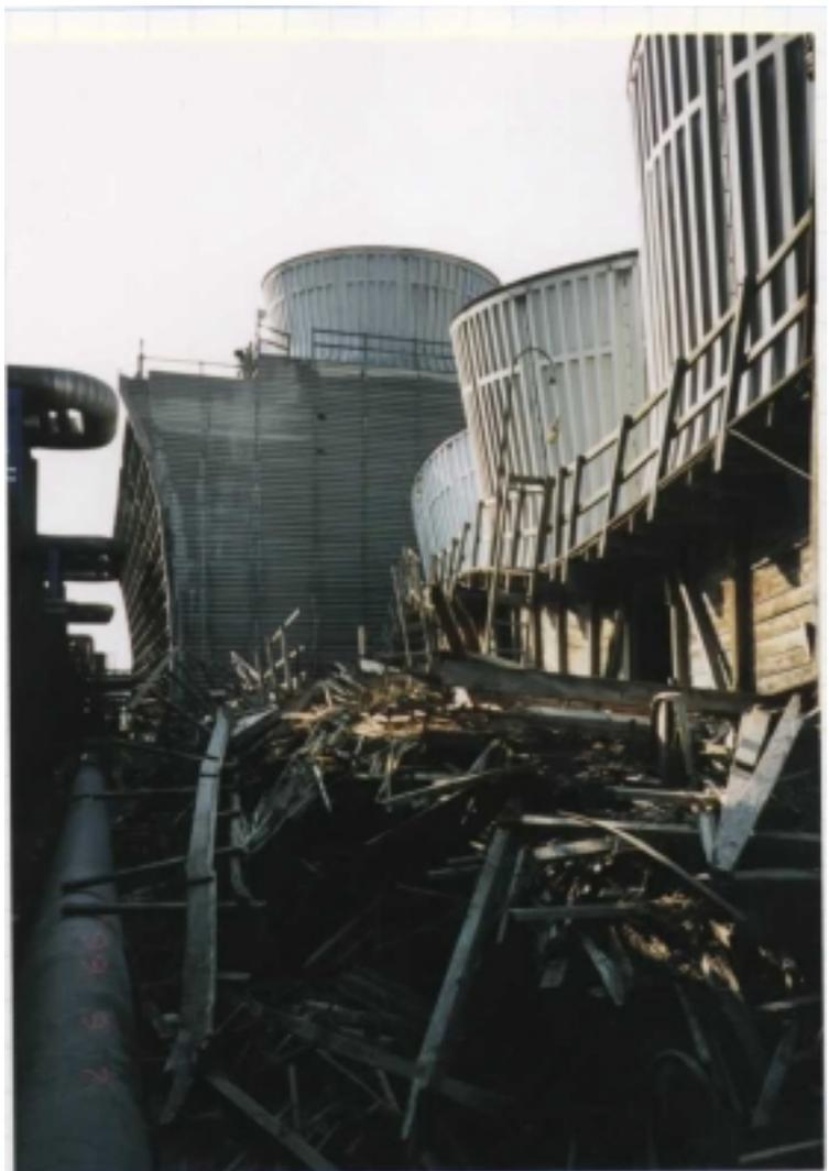
Figure 7.19 Collapsed wooden cooling towers (concrete
