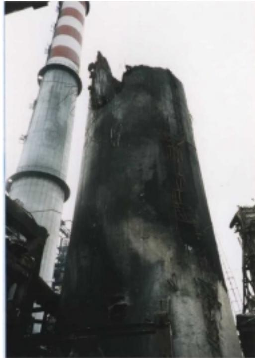
Figure 7.8 Collapsed stack
