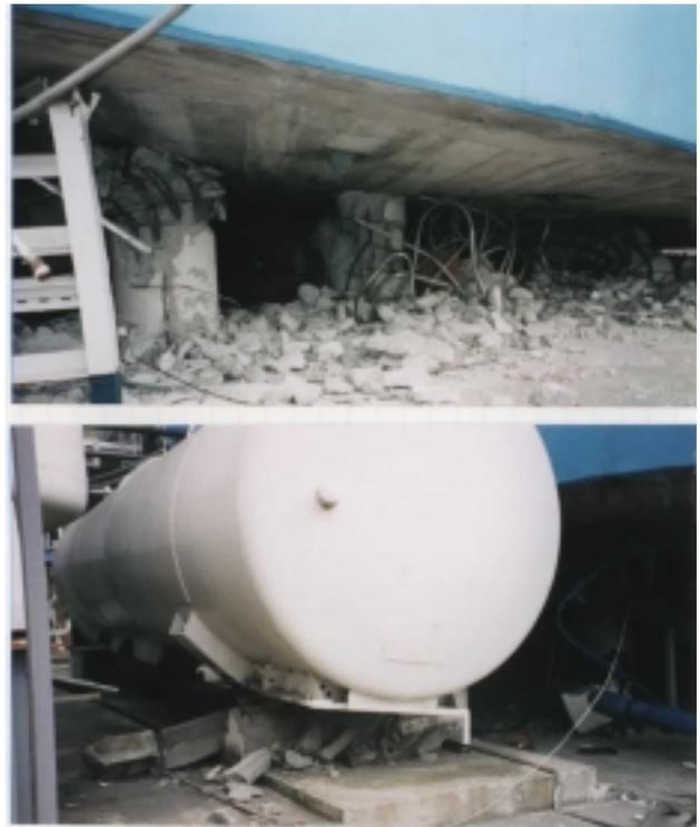
Figure 7.22 A close-up view of broken support columns of the vertical cylindrical tank and an adjacent horizontal cylindrical tank
