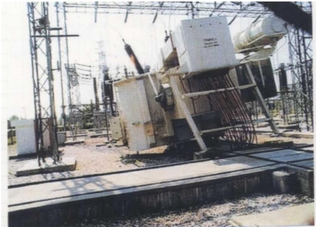
Figure 7.16 Fallen transformer (courtesy of TOYOTA-SA)
