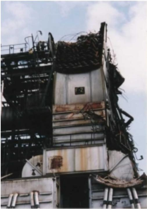
Figure 7.7 Damaged crude oil furnace
