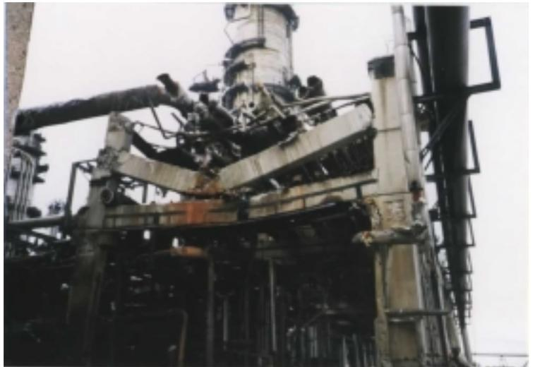
Figure 7.9 Damaged pipe-rack hit by the collapsed stack
