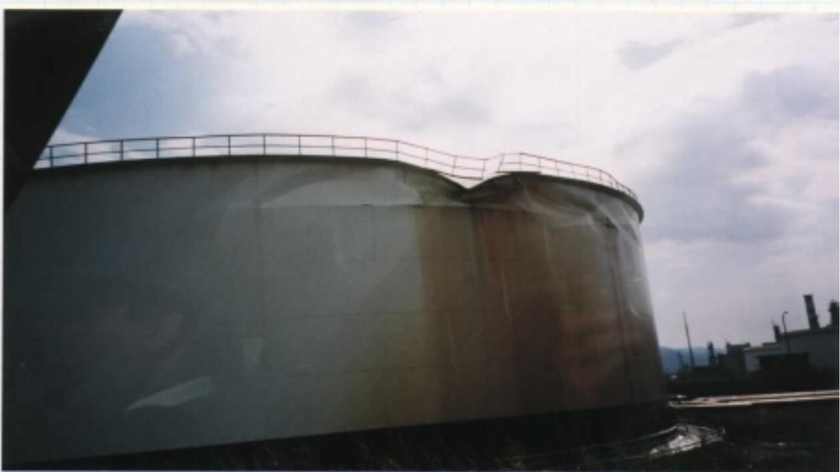
Figure 7.6 Deformation of a cylindrical tank with a fixed roof
