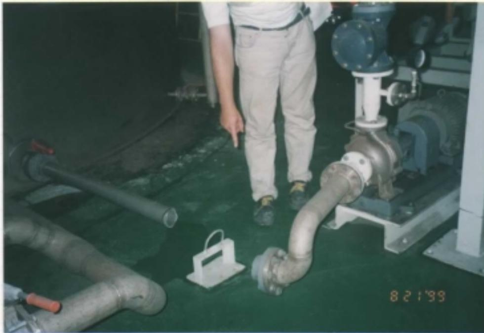
Figure 7.17 Sliding of Cooling water tank and rupture of pipes (courtesy of TOYOTA-SA)
