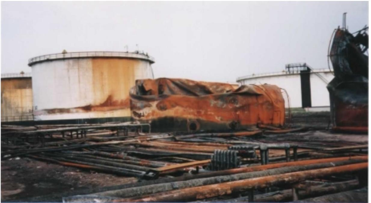
Figure 7.4 Burned cylindrical tank
