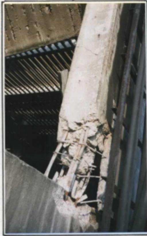
Figure 7.20 Damaged support columns of reinforced concrete towers
