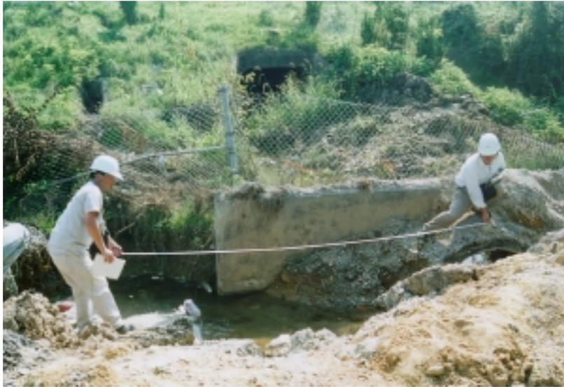
Photo 5.5 Offset of a Drainage Pipe of about 3.6 m (Point I, refer to Fig. 2)
