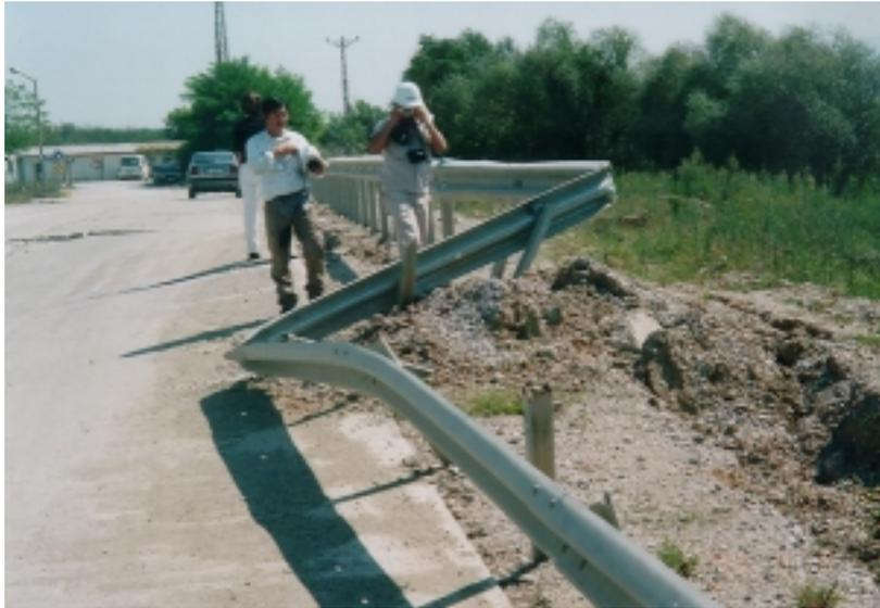
Photo 5.1 Damage of an Approaching Road to Toyota S.A. Factory (Point A, refer to Fig. 2)
