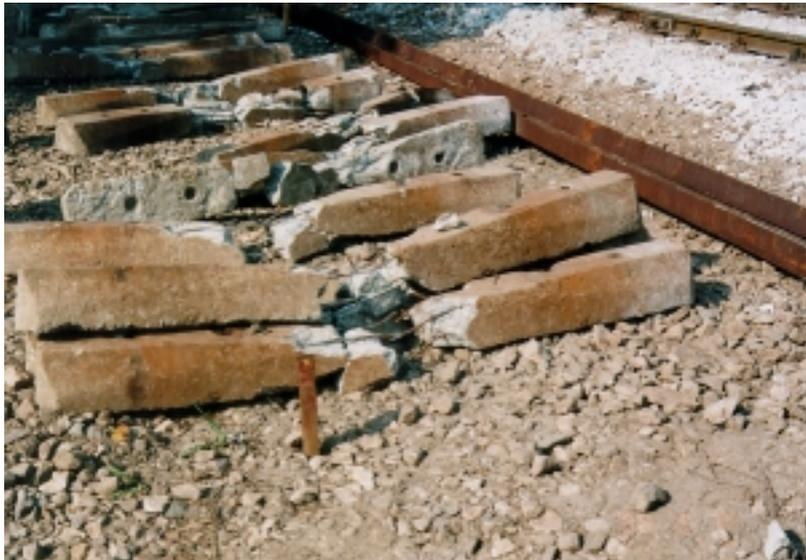
Photo 5.21 Damaged Rails and Sleepers, near Arifiye Overpass
