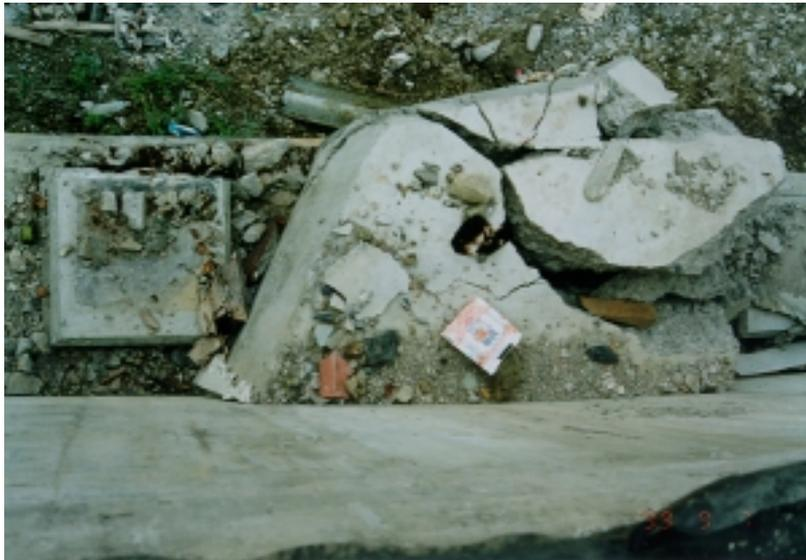
Photo 5.10 Damage of Reinforced Concrete Stoppers on A2 (Only west side was damaged), Arifiye Overpass
