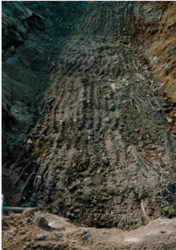
Photo 5.12 Piles That Supported P3 Footing, Arifiye Overpass
