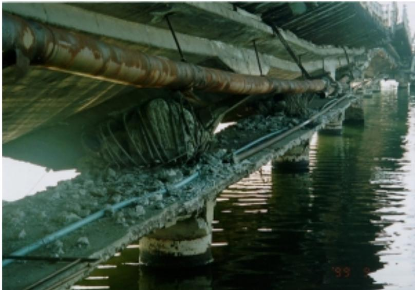
Photo 5.16 Shear Failure of Reinforced Concrete Columns
