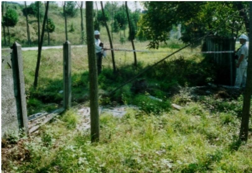
Photo 5.2 Offset of a Concrete Fence at of 4.3 m North-East Corner of an Automobile Factory (Arbas Arac Kadlama Fabzikasi) (Point D, refer to Fig. 2)
