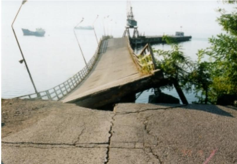
Photo 5.15 Damage of an Approaching Bridge in a Paper Factory
