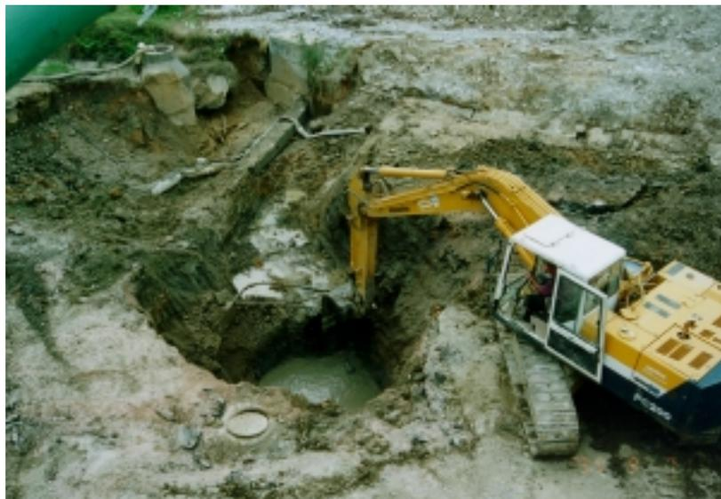
Photo 5.4 Offset of a Sewer Pipe of about 4 m (Point H, refer to Fig. 2)
