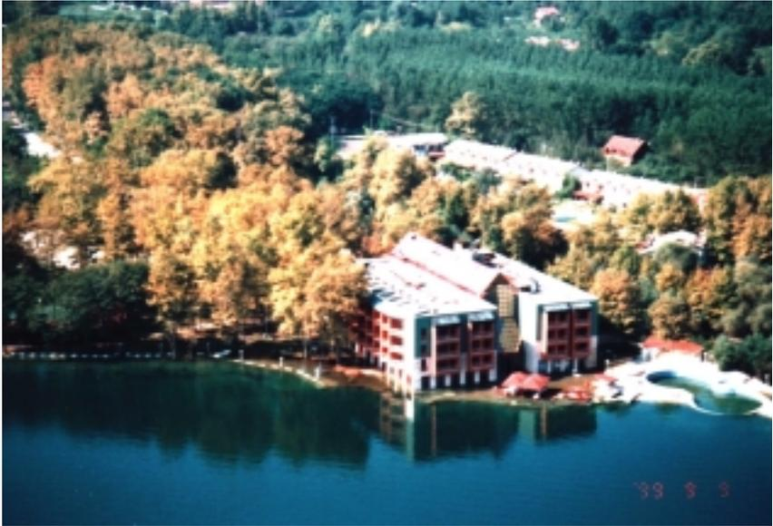
Figure 12.4 Lateral spreading and settlement of a hotel along the shore of Sapanca Lake (details of liquefaction site is shown in Figure 12.3)
