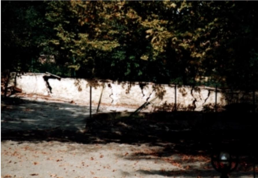
Figure 12.3 Wide-spread sand ejection and lateral spreading along souther shore of Sapanca Lake near Sapanca town (note the settlement and separation of the wall in the background)
