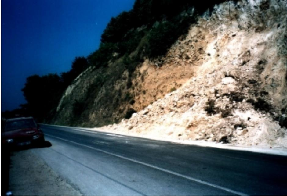
Figure 12.16 Rock slope failure at Kocaeli-Sakarya provincial boundary along D-100 highway (note that the car on the left-hand side of the highway was hit by the fallen debris)
