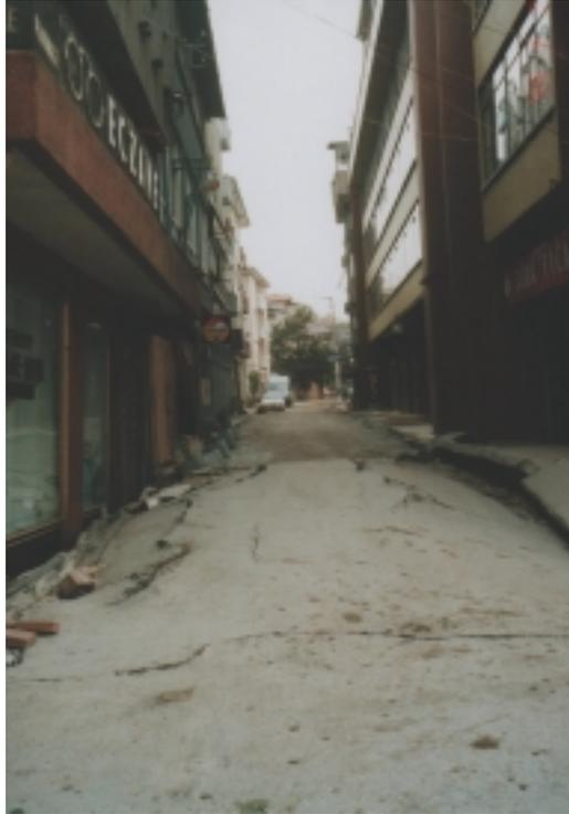
Figure 12.6 Heaving of a roadway as a result of settlement of adjacent buildings and the uplift of sewage pipe
