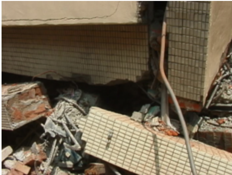
Figure 9.5. Collapsed columns and beams of the right building in Figure 4.
