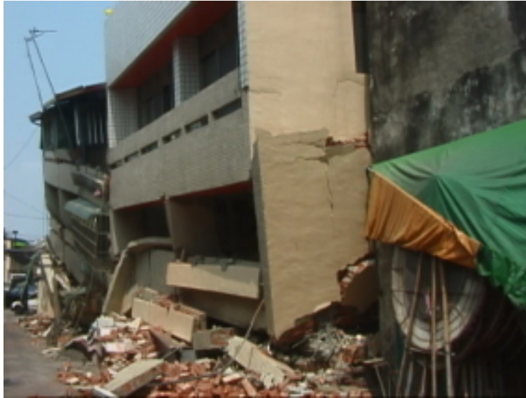
Figure 9.4. Damage to two 3-story RC apartment buildings in Nantou.
