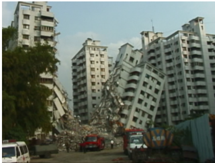
Figure.9.12. Damage to RC condominium buildings in Dali.
