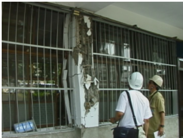
Figure 9.7. Collapsed column of the first story of the school building in Figure 9.6.
