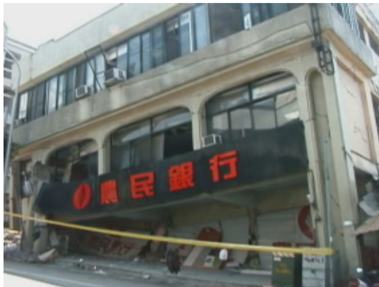
Figure 9.1. Damage to 3-story RC building in Ji-Ji.
