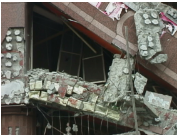
Figure.9.17. Collapse of a RC condominium building in Taichung.
