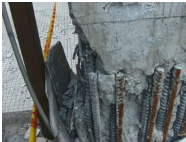
Figure.9.13. Broken column of a condominium building in Dali.
