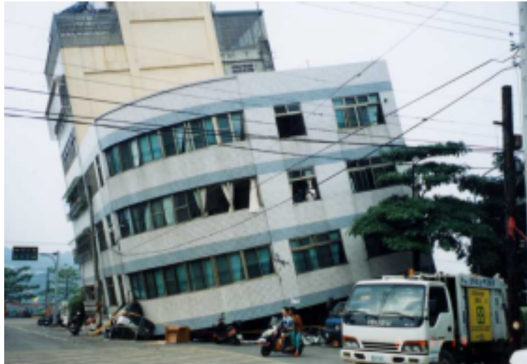
Figure.9.22. Collapsed 4-story RC building in Tungshe.
