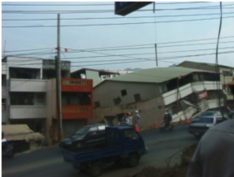
Figure.9.21. Collapsed building on a surface rupture in Fengyuan.
