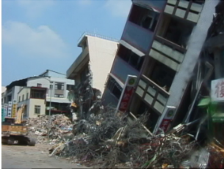
Figure.9.8. Damage to RC buildings due to differential settlements in Wufung.
