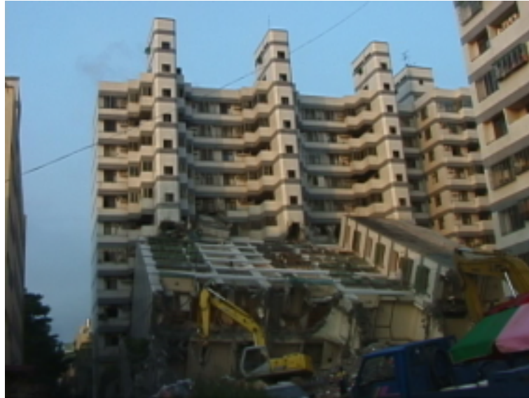
Figure.9.14. Damage to RC condominium buildings in Dali.
