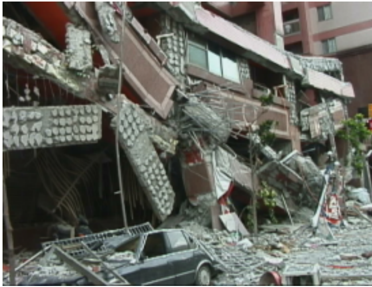
Figure.9.18. Collapsed beams of the building in Figure.9.17.
