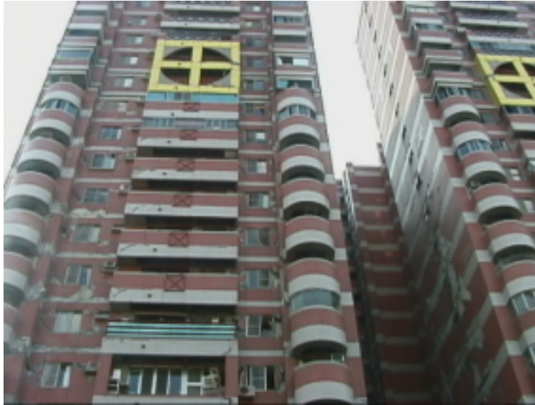
Figure.9.20. Shear cracks of a 22-story RC condominium building in Fengyuan.
