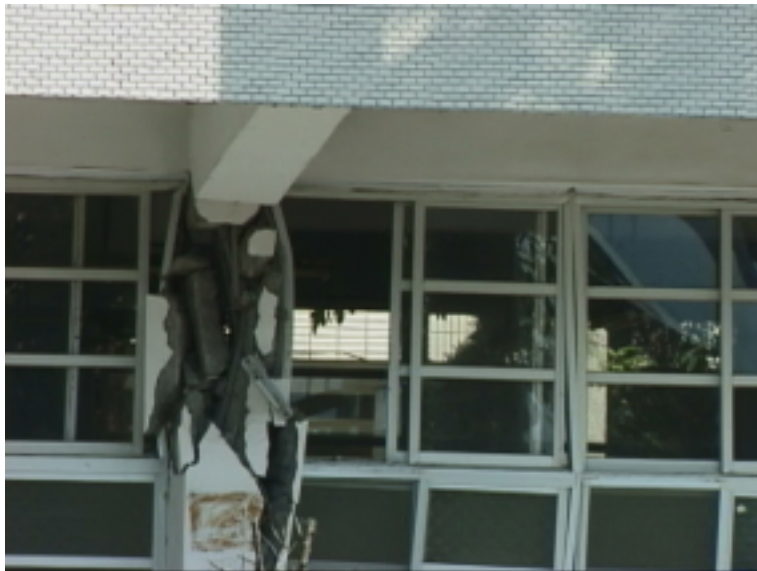
Figure 9.3. Shear cracks in a column of the first story of the building in Figure 2.
