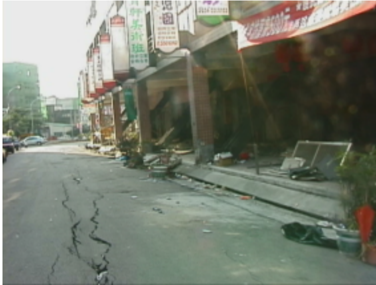
Figure9.10. Damage to the first story of the building in Figure 9.10
