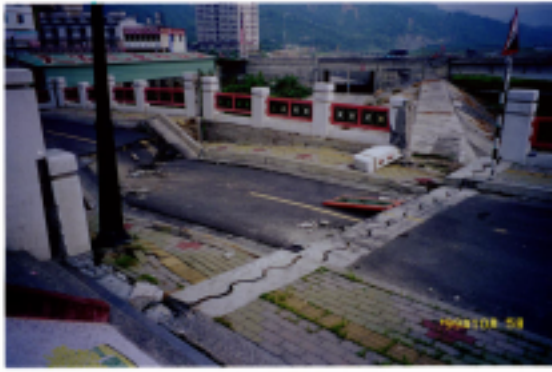
Photo.8.8 Failure of Abutment at Lyu-Mei Bridge(Provided from the investigation team for The 1999 Ji-Ji Earthquake by The Japanese Geotechnical Society)
