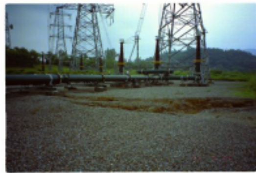
Photo. 8.13 Fissure generated by liquefaction
