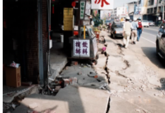
Photo.8.9 Settlement of Houses and Side walk
