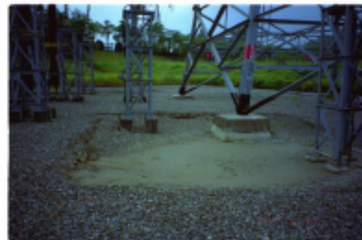
Photo. 8.15 Settlement of foundation of the transmission tower
