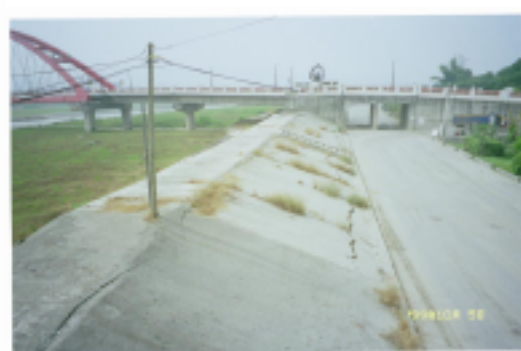
Photo.8.7 Crack along the facing of River Dike
