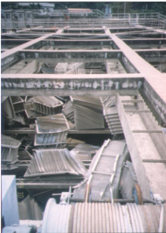
Figure.7.35 Damage at inclined plate clarifier (No.1 Fon-yuan purification plant)
