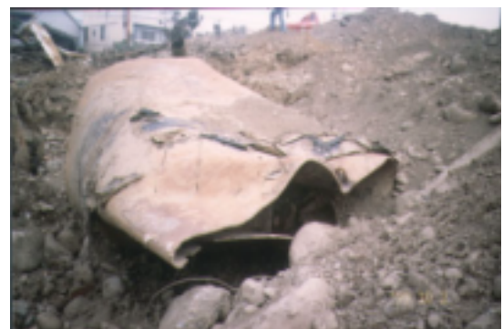
Figure 7.39 Damage to troughs at suspended solid contact clarifier (Rii-yui Tan purification plant)
