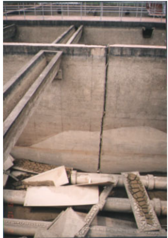
Figure. 7.34 Damage at suspended solid contact clarifier (No. 1 Fon-yuan purification plant)
