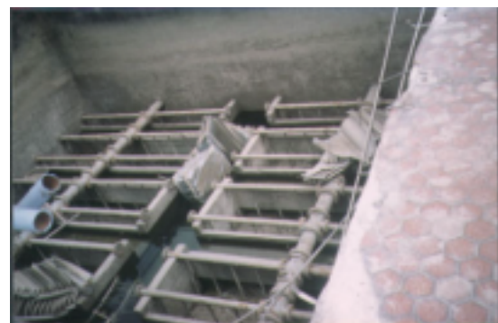
Figure.7.36 Jump out of inclined plates(No.1 Fon-yuan purification plant)
