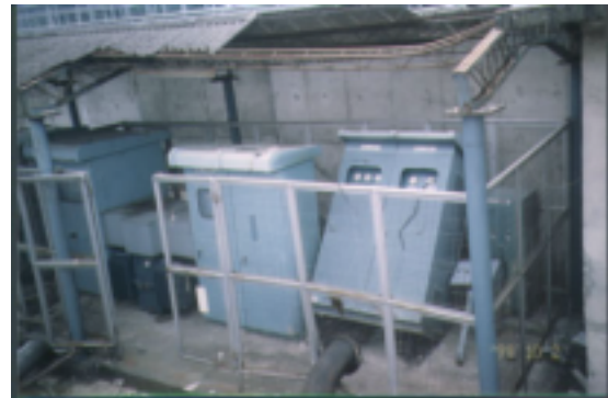
Figure 7.38 Overturn of control facilities(No. 1 Fon-yuan purification plant)
