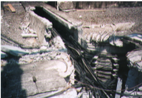
Figure 7.7 Damage of the Cable Ducts
