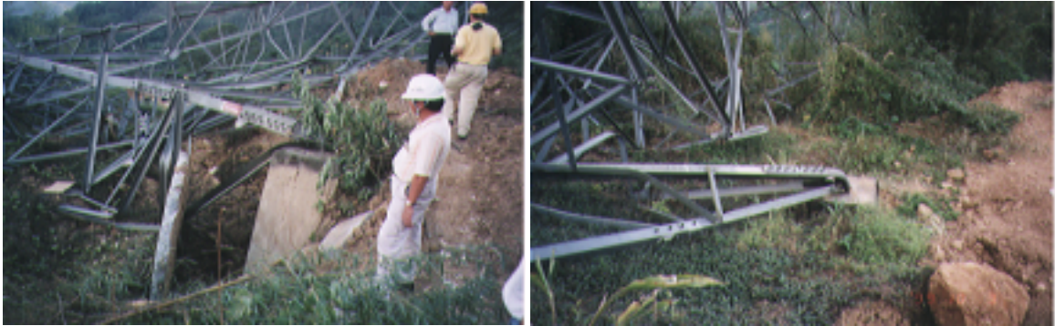
Figure 7.18 the collapsed tower # 203
