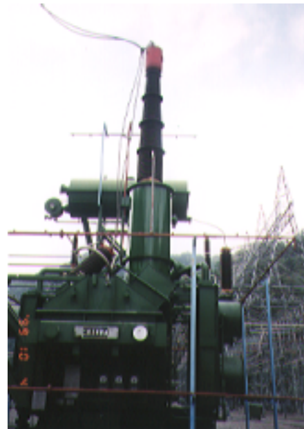
Figure 7.14 Damage of oil leakage at 345 kv Substation
