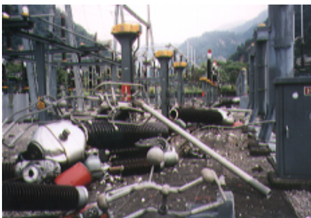
Figure 7.15 Damage of ACB at 345 kv substation
