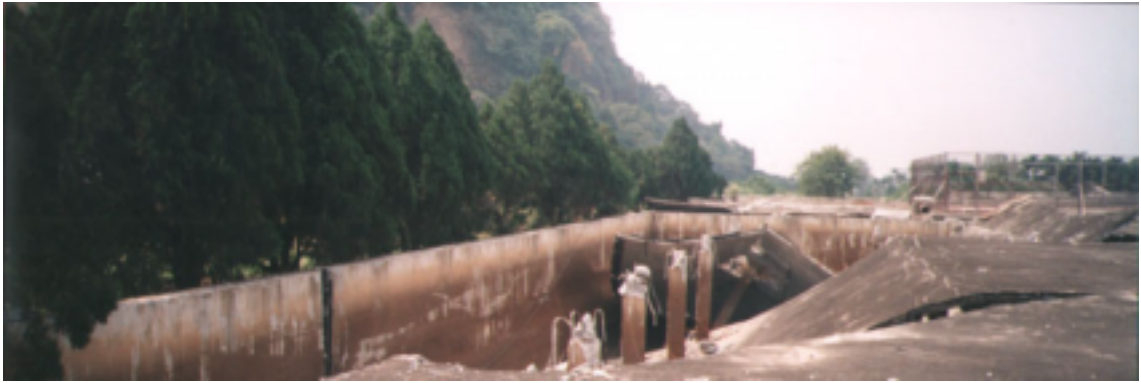
Figure. 7.37 Fall of ceiling slab of service reservoir (No. 1 Fon-yuan purification plant)
