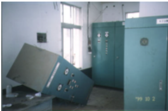
Figure 7.38 Overturn of control facilities(No. 1 Fon-yuan purification plant)
