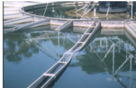
Figure 7.39 Damage to troughs at suspended solid contact clarifier (Rii-yui Tan purification plant)
