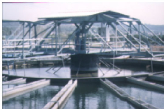
Figure 7.39 Damage to troughs at suspended solid contact clarifier (Rii-yui Tan purification plant)
