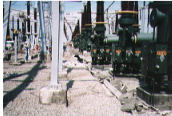
Figure 7.10 Ducts and GIS
