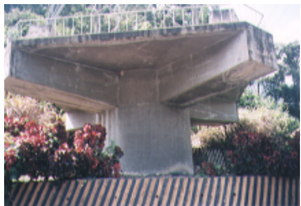
Figure 7.16 Well-type Tower Foundation
