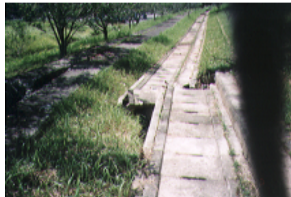
Figure 7.8 Damage of the Culverts
