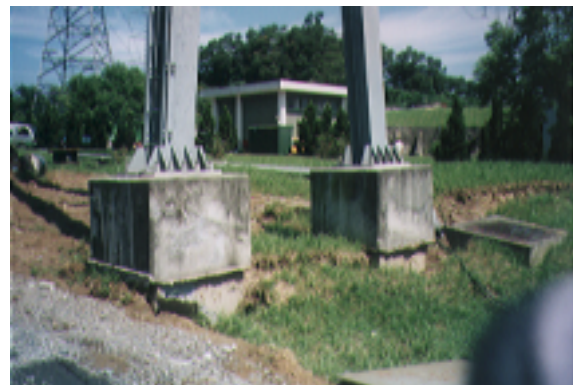
Figure 7.12 Damage of Foundation
