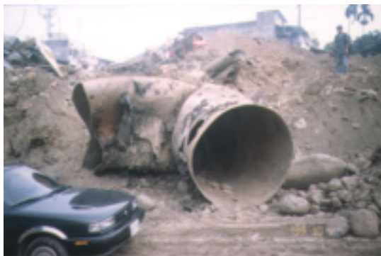
Figure 7.39 Damage to troughs at suspended solid contact clarifier (Rii-yui Tan purification plant)
