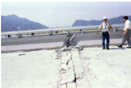
Photo 4.11 Pounding Failure of Girder
