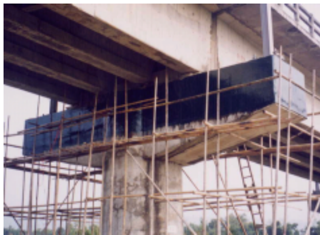
Photo 4.57 Reinforcement of projection part
