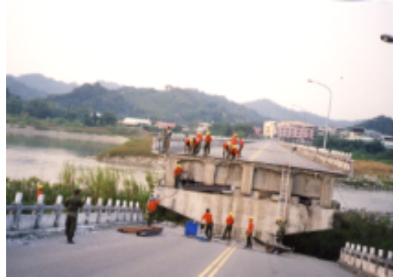
Photo 4.4 Failure pattern of CHANGGENG BIG Bridge
