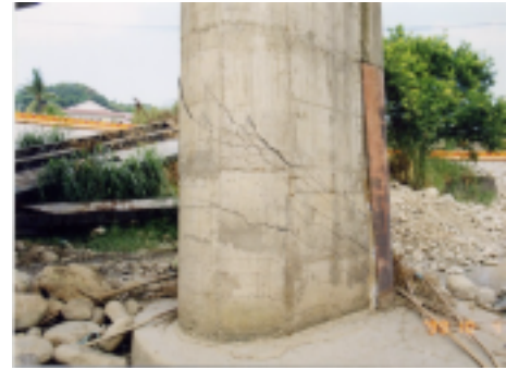
Photo 4.14 Damage of the pier
