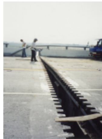
Photo 4.45 Gap at expansion joint
