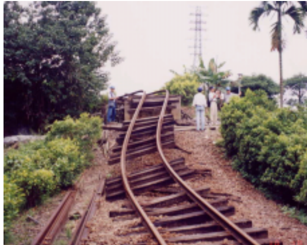
Photo 4.59 Damage in Chi-chi line (Mingchien)
