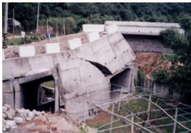
Photo.4.55 Damage of Underpass at Shishuikeng
