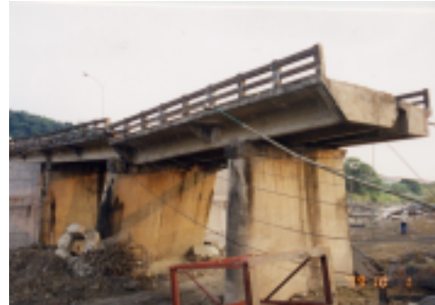
Photo 4.21 Shortened span
