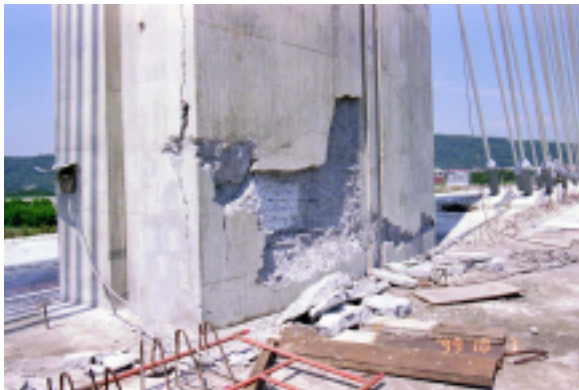
Photo 4.6 Cracks of Main Tower
