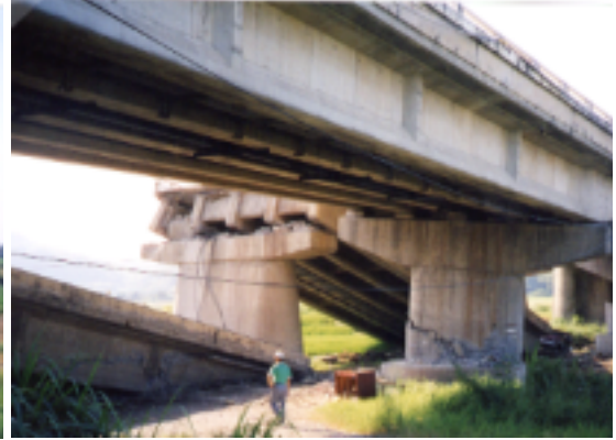
Photo 4.2 Shear failure of the wall-type pier
