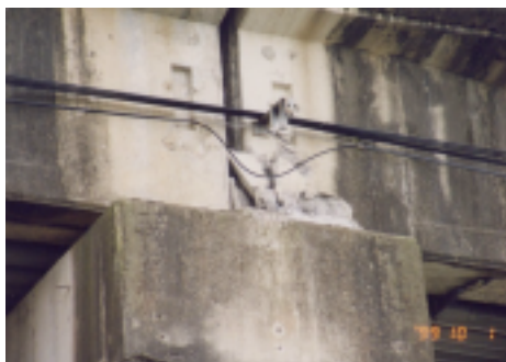
Photo 4.16 Damage at girder edge
