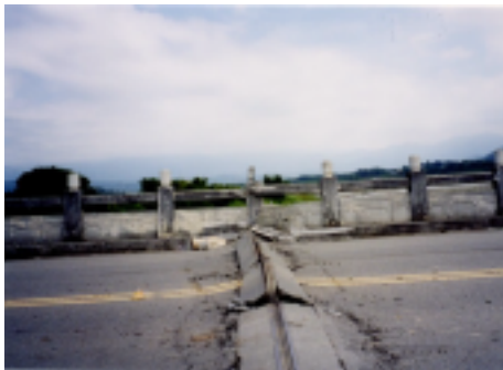
Photo 4.44 Compression of expansion joint
