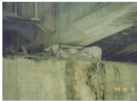
Photo 4.25 Bearing and side stopper
