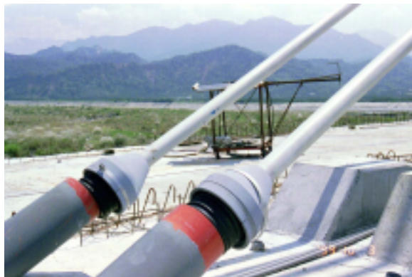
Photo 4.8 Pull Out of Cables (Damage Rank A)
