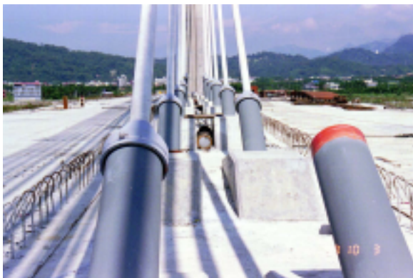
Photo 4.7 Breakage of Cable (Damage Rank As)
