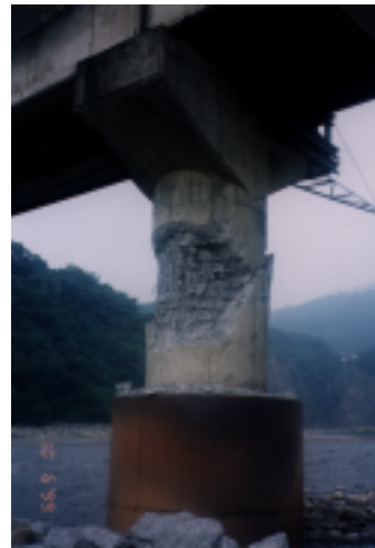
Photo 4.35 Damage of pier
