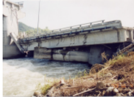
Photo 4.19 Collapsed substructure
