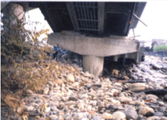
Photo 4.3 Failure of the Pier B4 of MINGZHU Bridge
