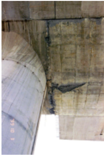
Photo 4.9 Buckling of Reinforcement
