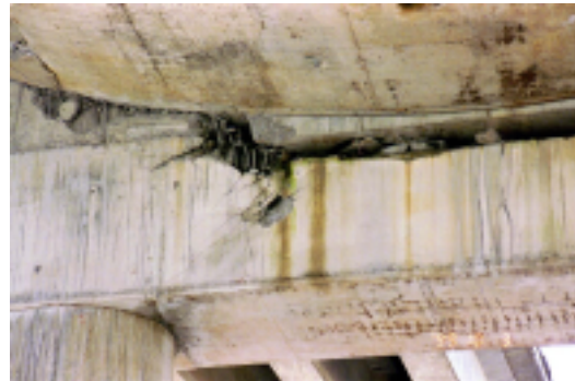
Photo 4.10 Shear Failure of Rigid-Frame Pier
