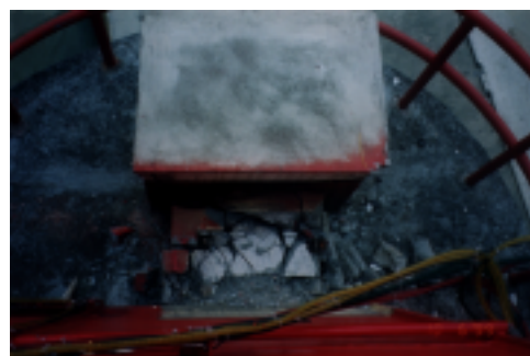
Photo 4.31 Failure of bearing
