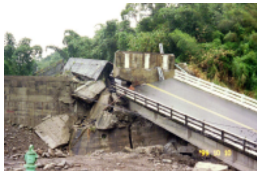
Photo 4.41 Collapse of Abutment
