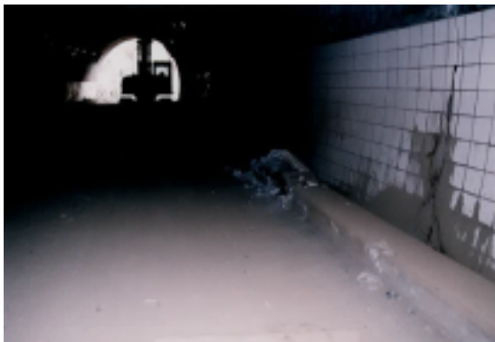
Photo.4.53 Damage of Side wall at Ma Ling No.2 Tunnel(Taiwan Road No.8)
