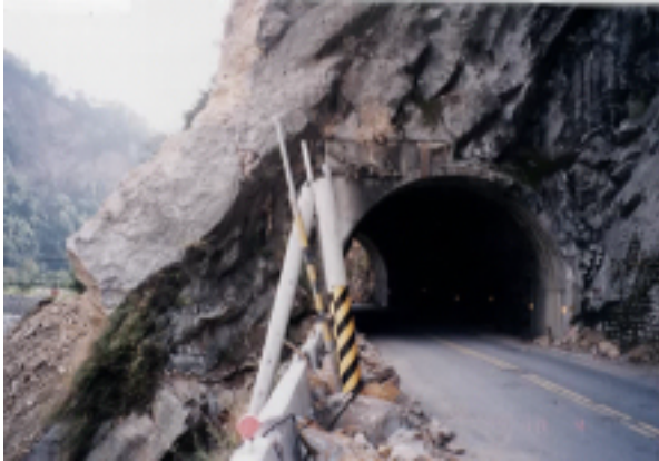
Photo.4.51 Damage of Li Leng Tunnel (Taiwan Road No.8)
