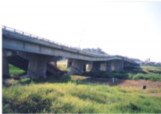
Photo 4.1 Failure pattern of WU-SHI Bridge
