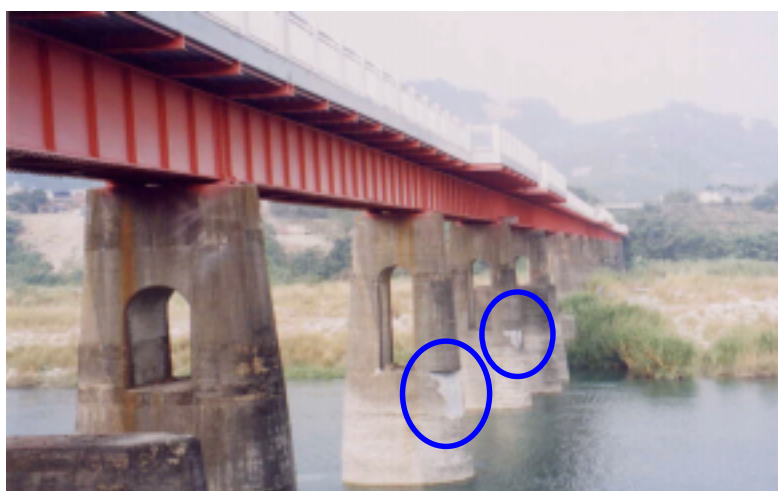
Photo 4.64 Damage of old railway bridge
