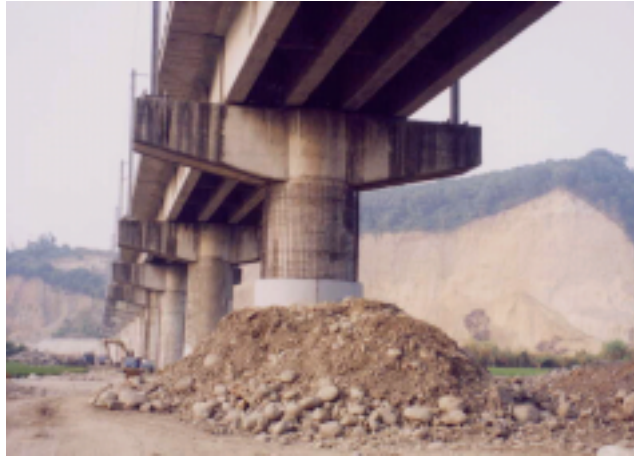
Photo 4.56 Reinforcement of elevated bridges
