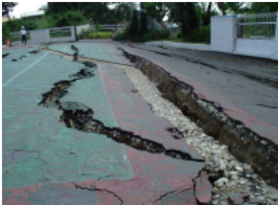
Photo3.12 The appeared fault with NS strike on the pavement ground
