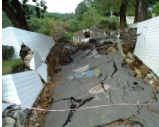
Photo3.12 The appeared fault with NS strike on the pavement ground
