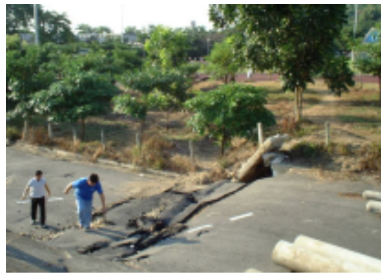
Photo3.14 A small horizontal displacement is recognized
