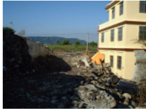
Photo 3.5 Movement of the house by the landslide
