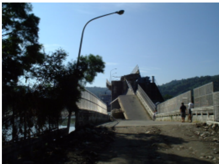
Photo 3.7 Uplift of floodgate ( 9.8 m) and right-bank abatement (2 m)
