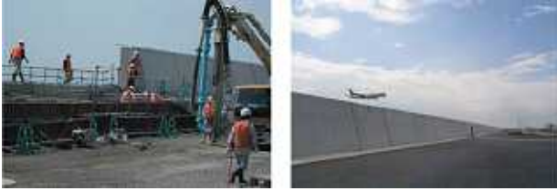
Photo 3. Construction work to raise the seawalls (left); completed seawall (right).
