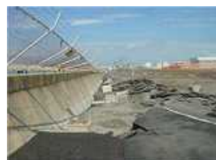
Photo 2. Seawall damaged by high waves (damage caused by Typhoon 16 of 2004).
