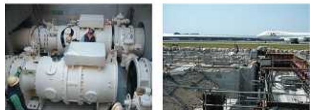
Photo 1. New, improved horizontally oriented underwater pump (left); pump pit construction next to the runway (right).
