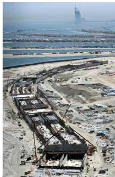
Photograph 2. Work on the undersea road tunnel.
