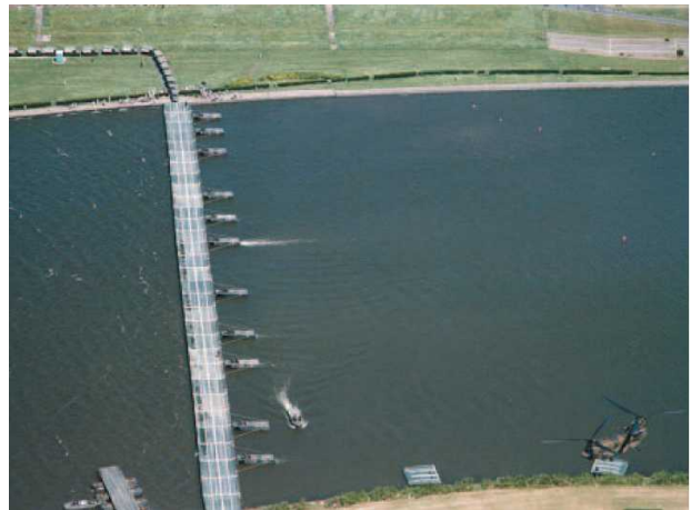
Photo 4. A heavy pontoon bridge installed by the Ground Self-Defense Forces in a few hours' time (Edo River).
