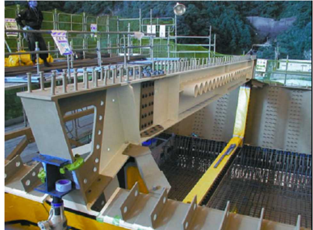
Photo-5: On-site assembly of steel diaphragm
