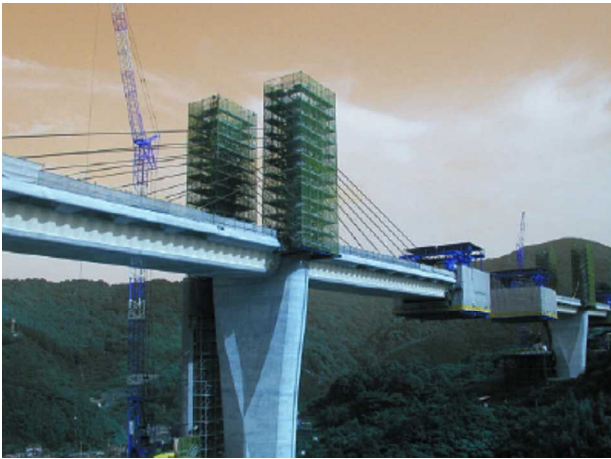
Photo-4: Cantilever erection method by a traveler
