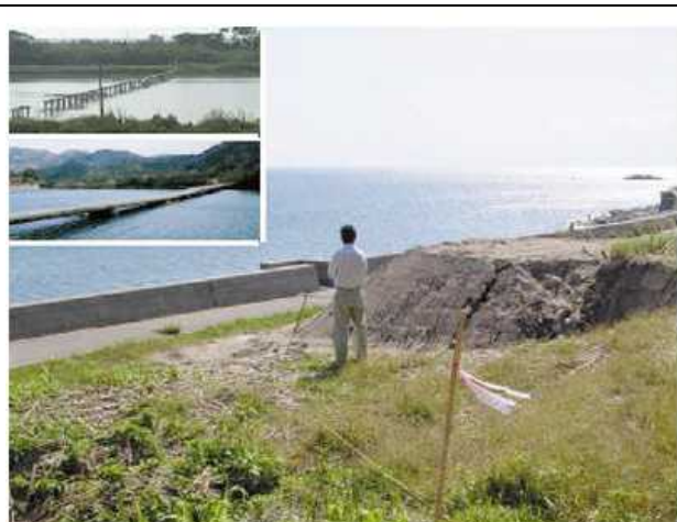
Photo-2 The left top is a flow bridge, the bottom is a submerged bridge. The girders of these bridges are drifted or submerged when the water rises, they come back easily when the water level lowers. These are typical of early evacuation models.
