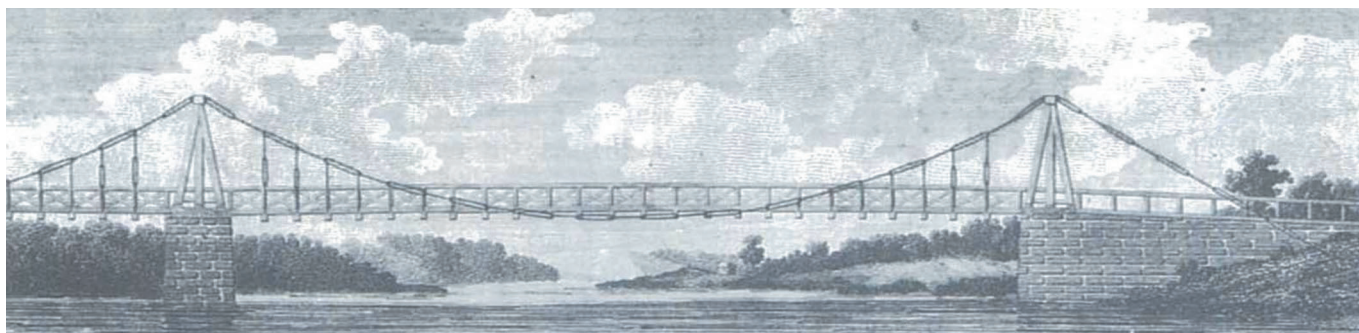
Figure-1: Patent James Finley: With the added stiffening girders, this bridge is an early model of modern suspension bridges.
