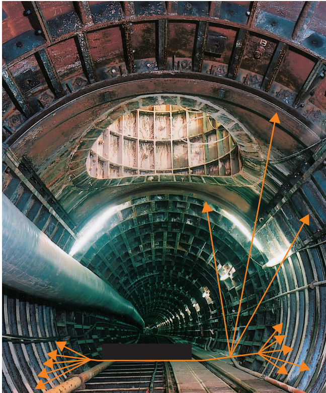
Photo-3: The primary lining completion
