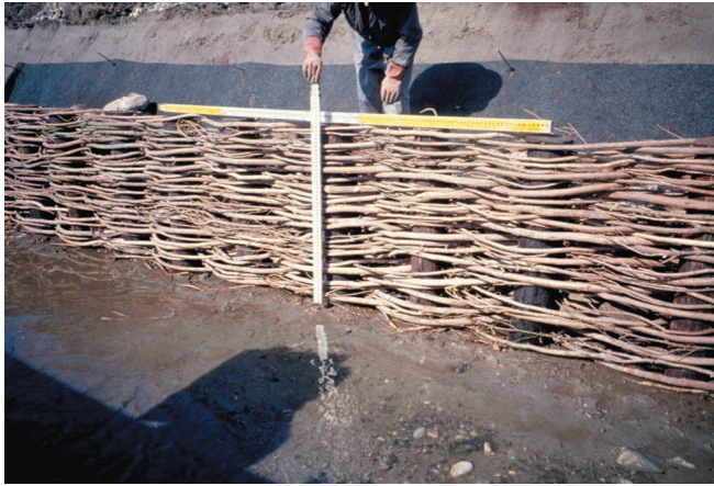
Photo-2: February 1994 Soda revetment h=one-meter)
