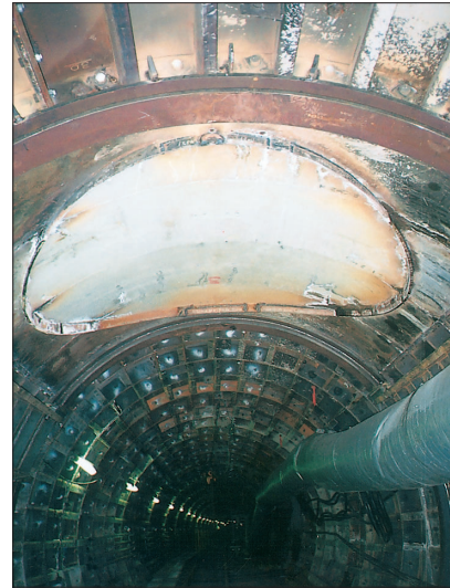
Photo-2: Opening segment installation
