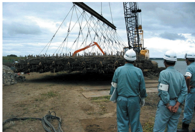
Photo-1: Hanging Soda mattress using a large crane
