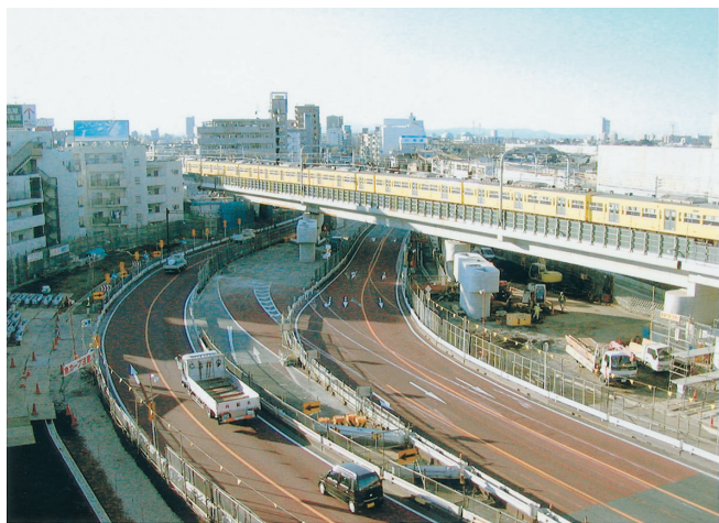
Photo-1: Reverse-multi-level crossings construction for the Seibu Ikebukuro Line.
