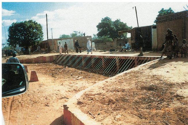
Photo-1: Drainage along the road and the protection screen
