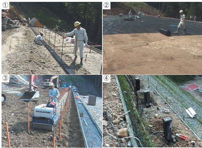
Photos-3: ①Reaction board, ②Placement of Geogrids, ③④Compaction of the slope area.
