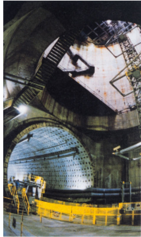
Photo 3 Umezato launch shaft and underground tunnel-shaped regulation pond
