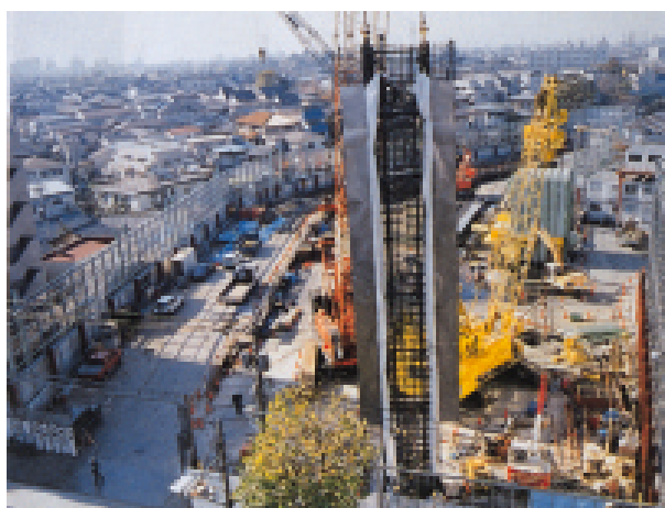
Photo 6 Cast-in-situ diaphragm wall under construction
