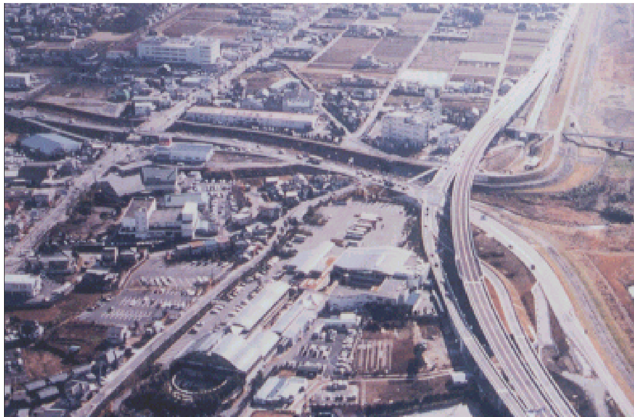
Photo 1 Aerial view of Ohito Viaduct
