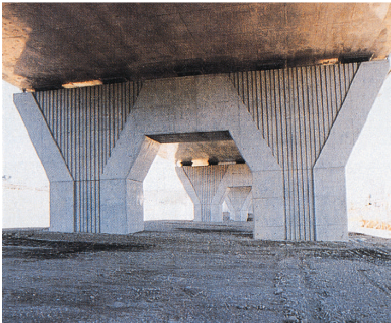
Photo 2 No. 2 viaduct pier
