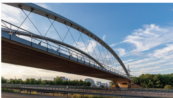
Fig. 3 A Network Arch Bridge with carbon hangers [3].
