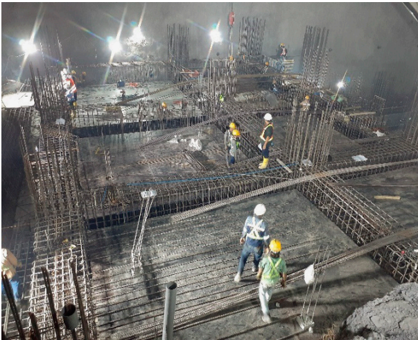
Install Rebar Election bay EL=68.7
