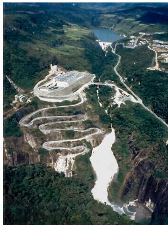
Photo 4: Panoramic View of Power Plant No. 1 (Siguragura Dam)
