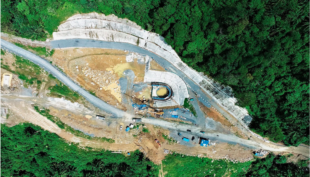
Headpond Shaft Concreting Works and Detour Roadworks
