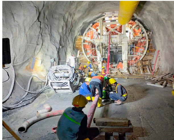
Installation of Concrete Delivery Pipe
