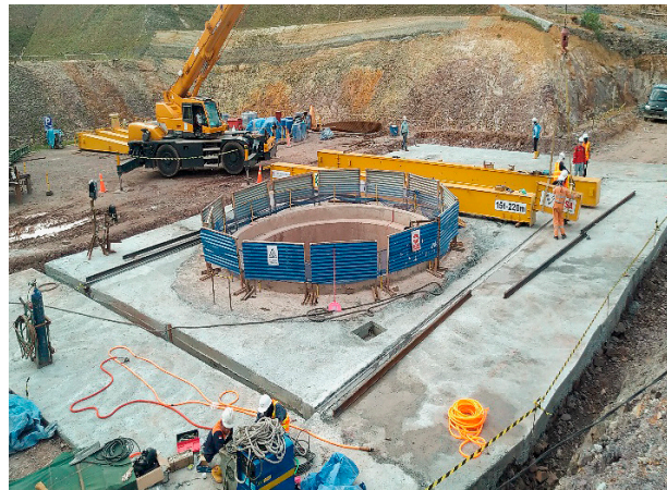
Gantry Crane Assembling
