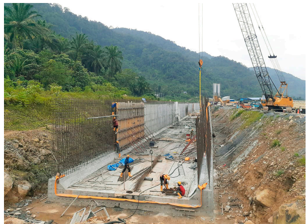
Structure Work Sta.1+000 – 1+260
