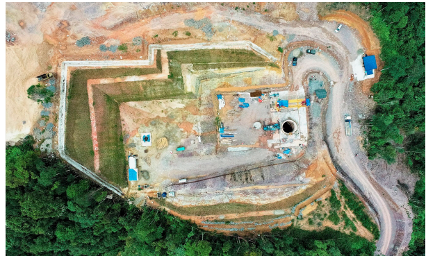
Installation of Gantry Crane & Penstock Inspection Shaft Excavation
