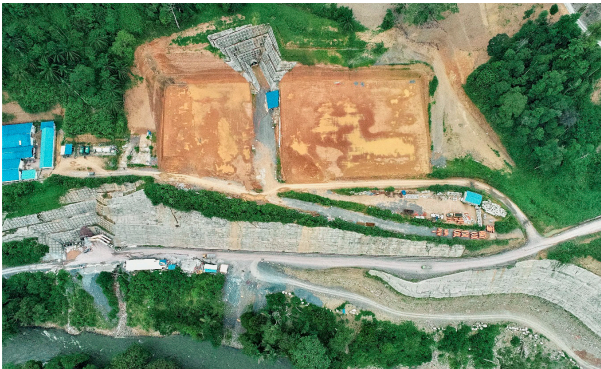
Hauling Material to Spoil Bank No. 6
