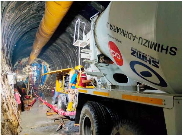
Placing lining concrete
