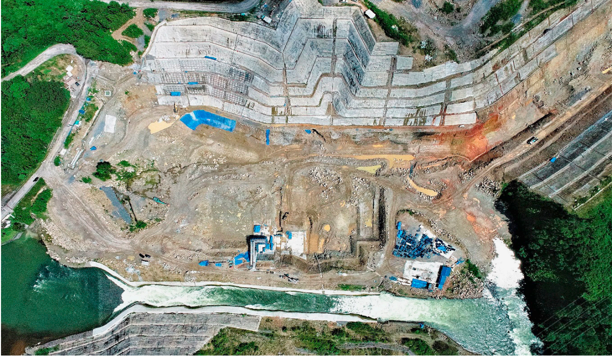
Excavation at Intake Facilities & Intake Weir Concreting
