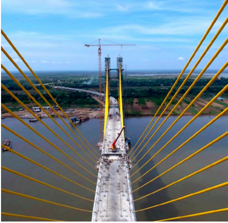
Photo 7: View of the West Side from the East Main Tower
