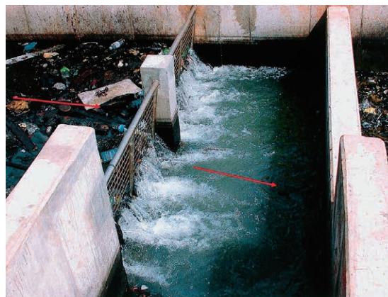
Photo 4: The refuse is removed at the screen
