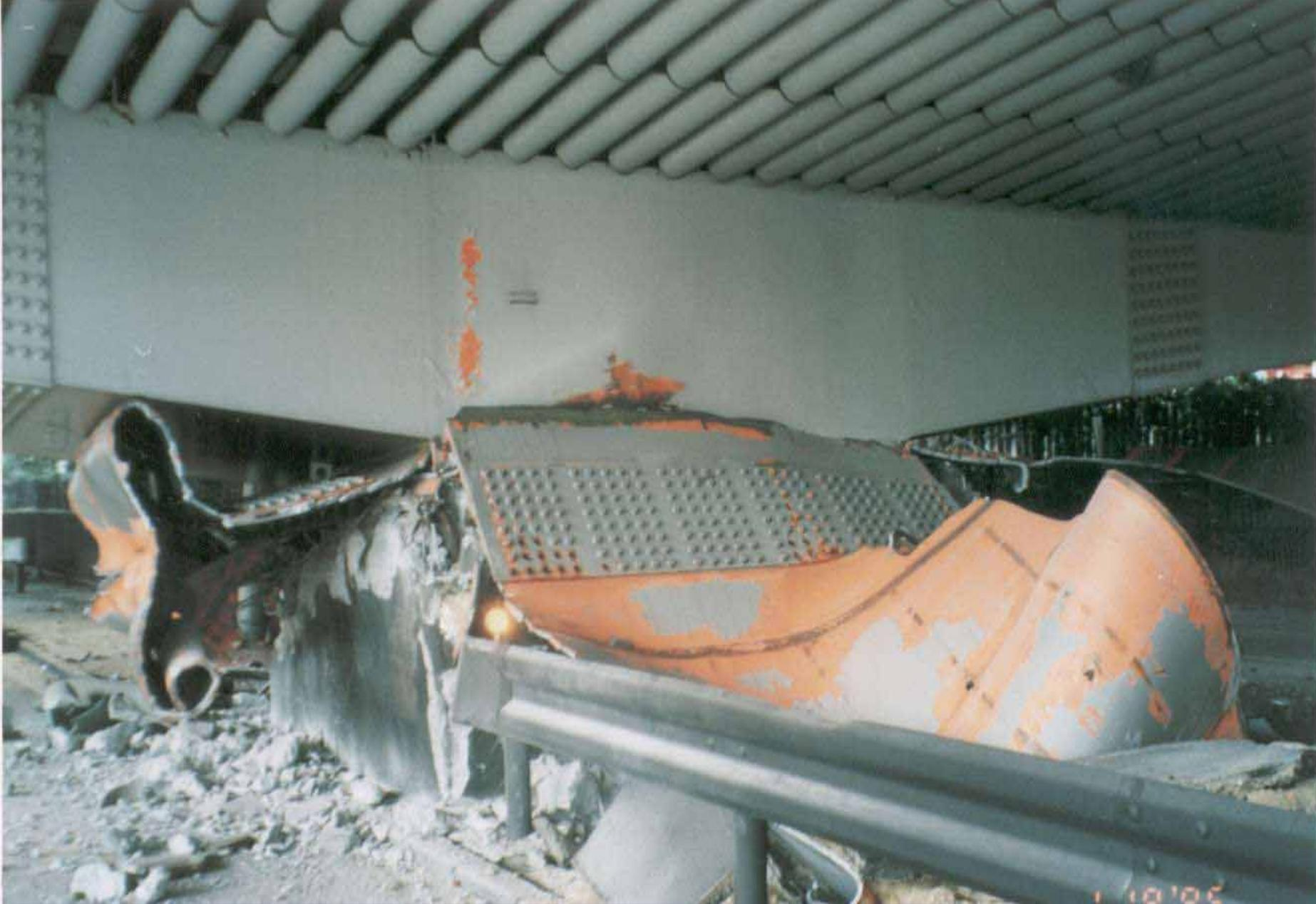
**Failure of Steel Box Pier due to Corner Weld Rapture**
