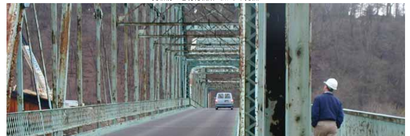
Ford City Bridge, PA
