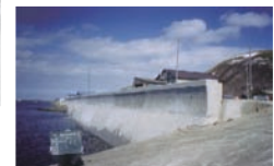
The revetments after corrective measures, with anterior embankment widening.
