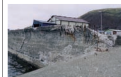
Prior to corrective measures, these revetments were in a dilapidated state with deteriorating concrete.
