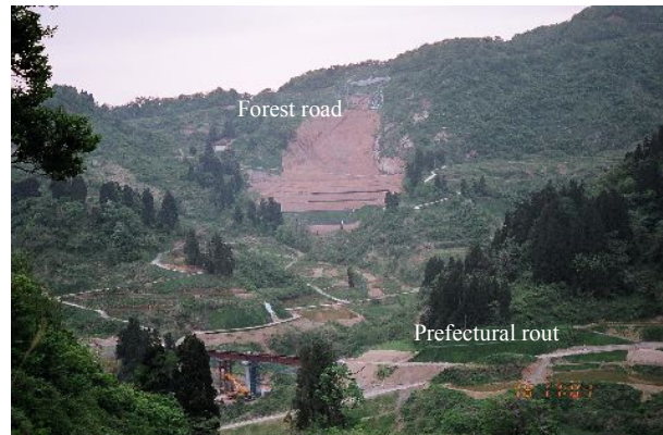
Restored roads and stabilized slope in Kazeguti pass
