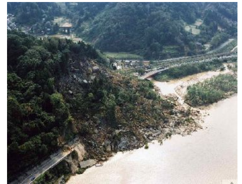
A view of the collapse situation from the sky over northern side (Offered by Niigata prefecture)
