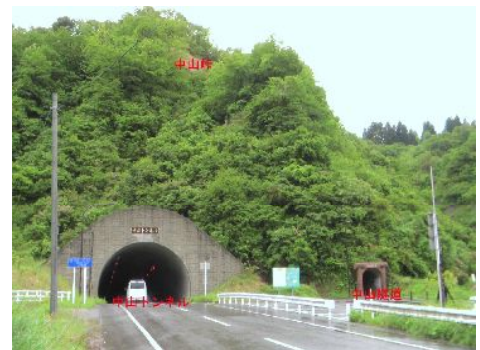
New Nakayama tunnel and old Nakayama tunnel where constructed by hand-excavate
