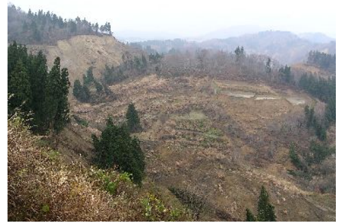
The cliff of left side were occurred by movement of soil mass
