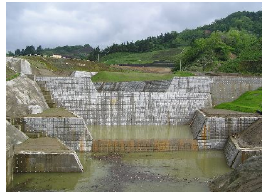
Behind the Sabo dam is a stabilized slope where soil mass were cleared
