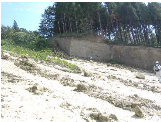
Slipped surface as smoothly (The mark of collapse) and rock layer remained at the side of the collapse
