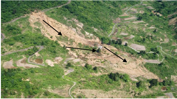
The weathered rock layer collapsed in upper part, the lower part was an old landslide (The arrows indicates the direction where unstable mass moved) (Offered by Forestry agency)
