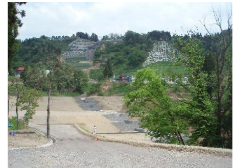
Stabilized slope in Takezawa and restored Yubu river
