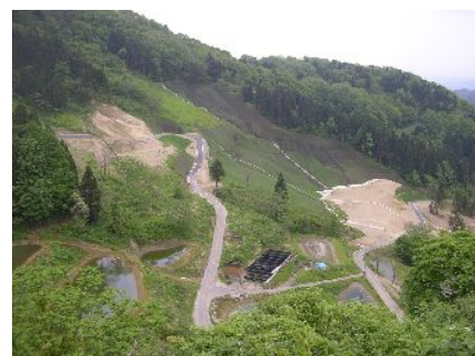
A view of the stabilized slope
