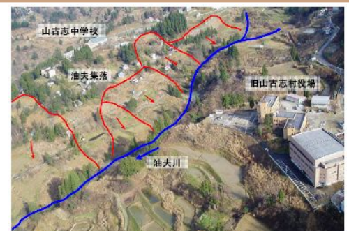
Landslide of Yubu River from sky over (Offered by Niigata prefecture)
