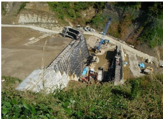
Sabo dam in downstream of land slide area of Terano
