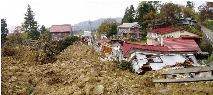
Collapsed houses by Landslide (Offered by Niigata prefecture)
