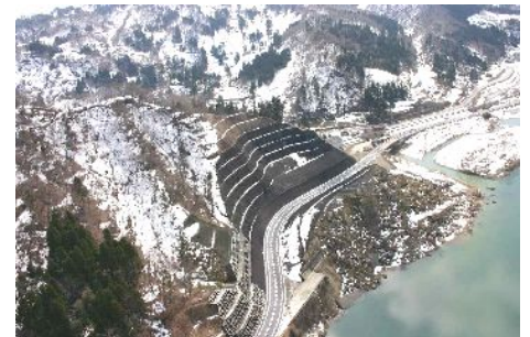
Stabilized slope and restored road (Offered by Niigata prefecture)
