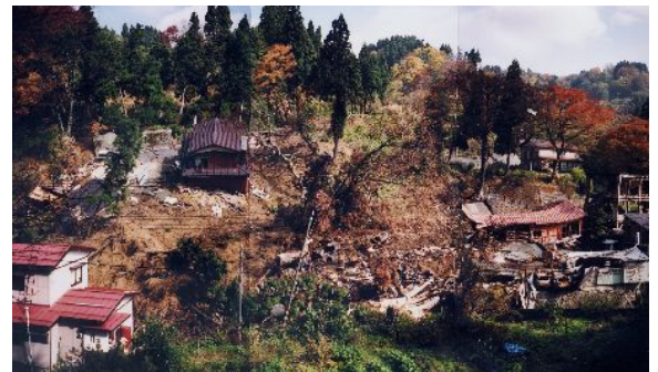
Collapsed houses by landslide
