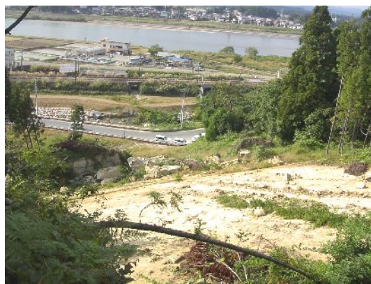
A view of the collapse situation and restored road from upper side of slope
