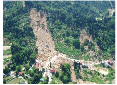
The large slope failure near the Haguro tunnel (left side) (Offered by Forestry agency)
