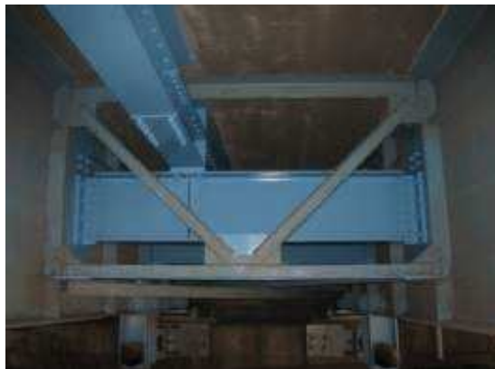
(a) 縦桁・横桁補強 Installing girders
