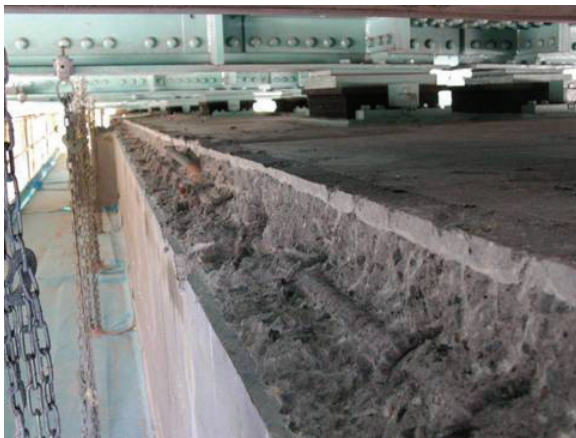
Photo 2.1 - Pier Beam Chipping Inspection
