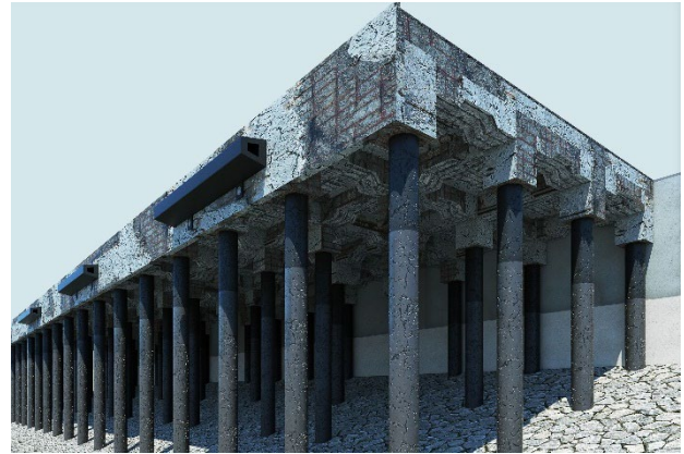
Figure 1. Port pier deteriorated due to reinforcing steel bar corrosion
