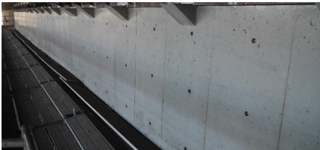
<Heat resistance> Repair of reinforced concrete retaining wall
